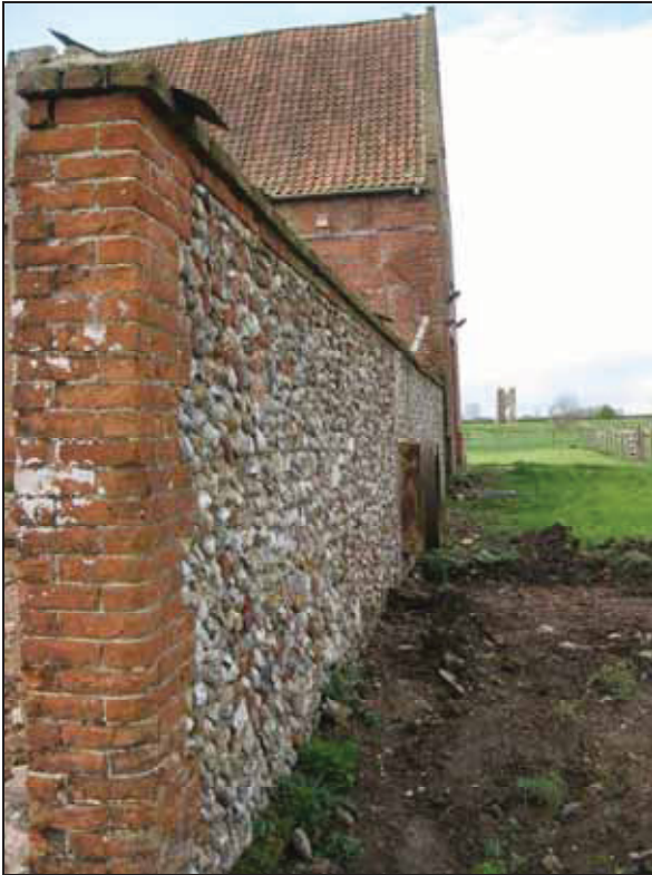
7 Surviving north wall of 18 th /19 th century extension. Looking west.
