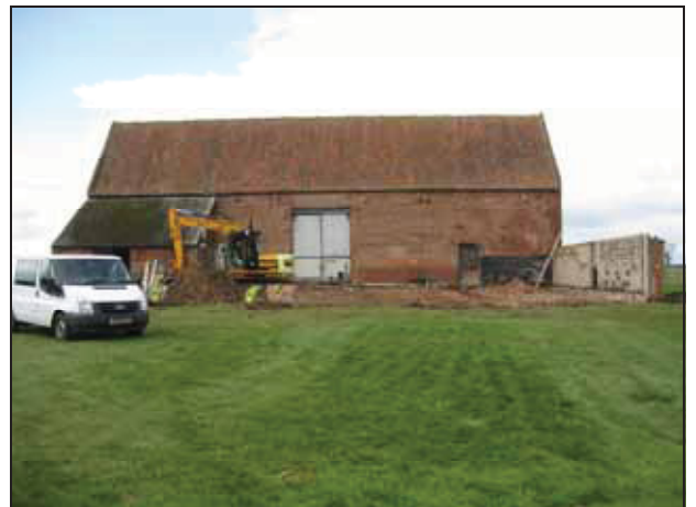
6 The Great Barn and the site. Looking west.
