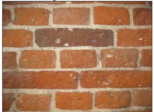
10 Late 16 th century brickwork within the barn.
