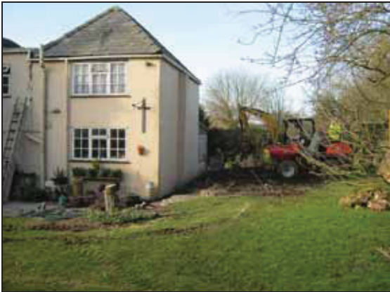
Work commencing to rear of Tannis Court House. Looking west.
