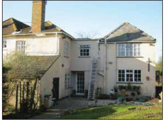
Rear of Tannis Court House. Looking west.
