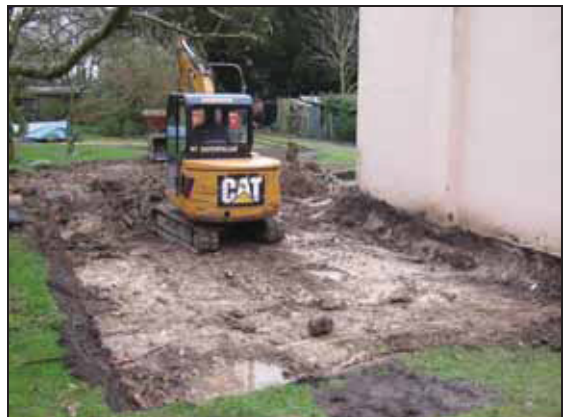
Post excavation view of extension footprint. Looking east.
