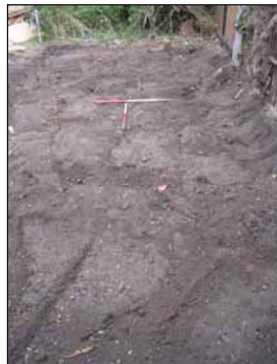
6 Ground reduction across garage footprint. Looking North-East
