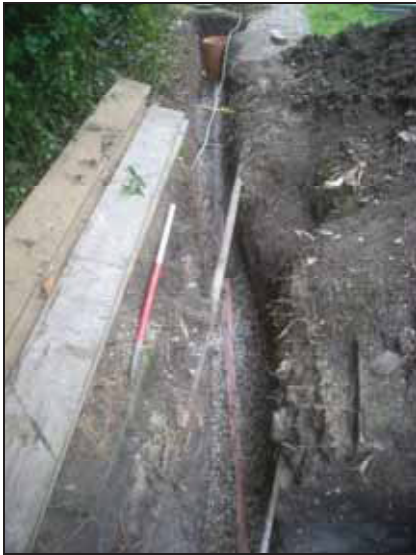
1 SW/NE arm of drainage trench. Looking North-East
