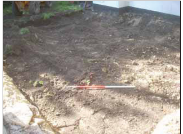
4 Ground reduction across eastern extension. Looking South-West
