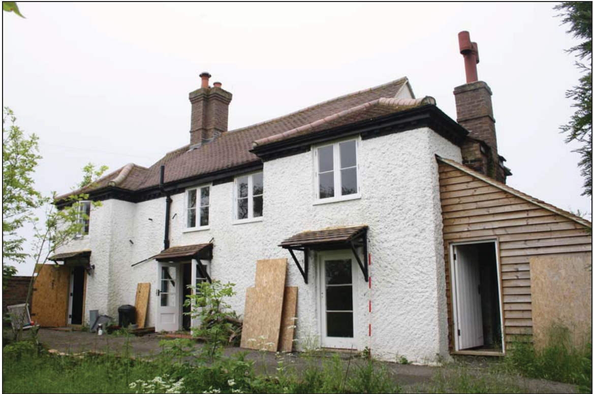
Plate 1 East elevation, taken from the north-east (DP 1)
