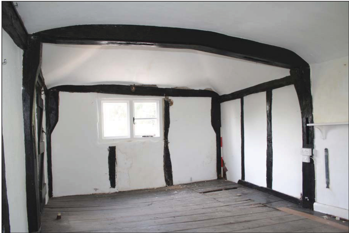
Plate 9 West side of Room FF05, taken from the east (DP 28)
