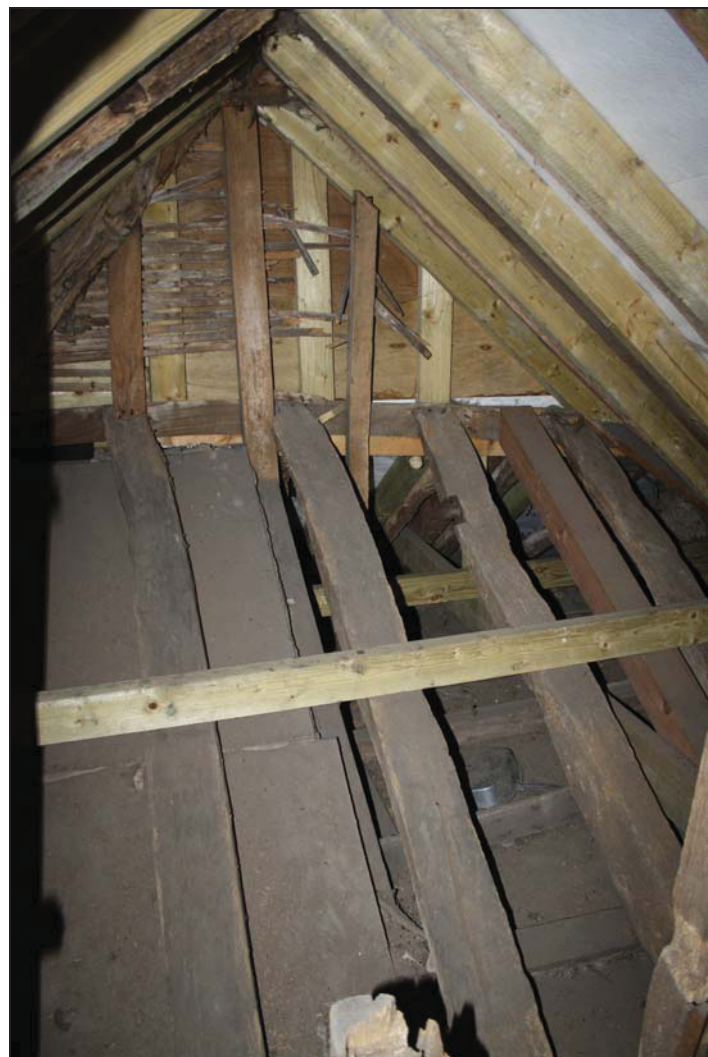
Plate 10 View of the roof over the northern cross-wing showing early repositioned rafters, taken from the south (DP 32)
