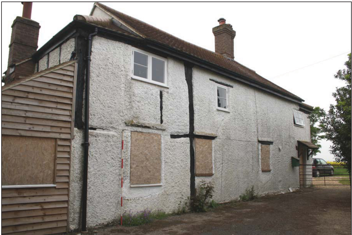
Plate 2 West elevation, taken from the north-west (DP 6)
