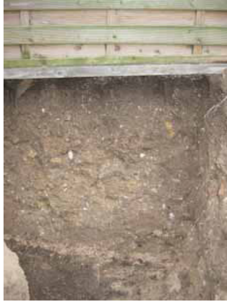
Post-excitation photograph of footings, Sample Section 2, looking south-east.
