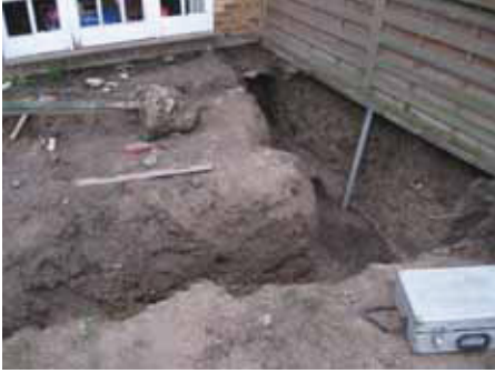
General site photograph, conservatory footings, looking north-east.
