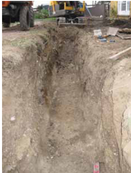
Excavated conservatory footings, looking north-west.
