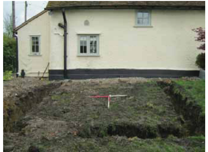
Foundation trenches for the extension, looking west.
