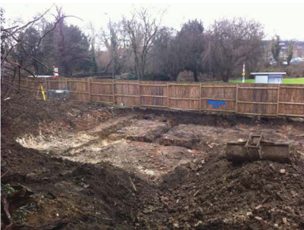
DP 5. Area 1. Foundation trenches. Looking west-south-west.
