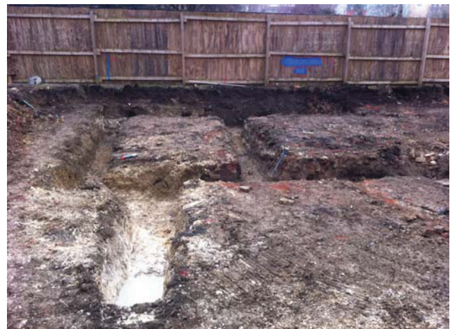
DP 6. Area 1. Foundation trenches. Looking west.
