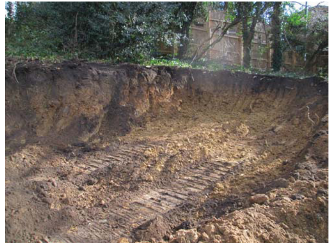
DP 2. Area 1. Excavations for a new soakway. Looking south-east.
