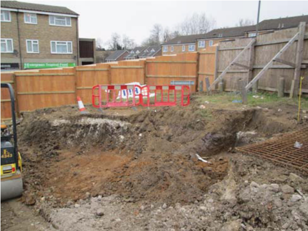
DP 13. Area 2, north-eastern corner. Looking north-north-east.
