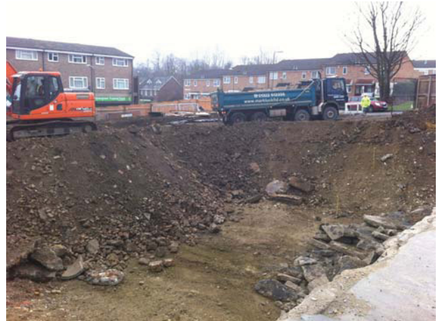
DP 16. Area 2. Looking north-east.
