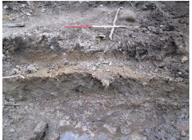
DP 10. Area 1. Foundation trenches, sample section 4. Looking west.
