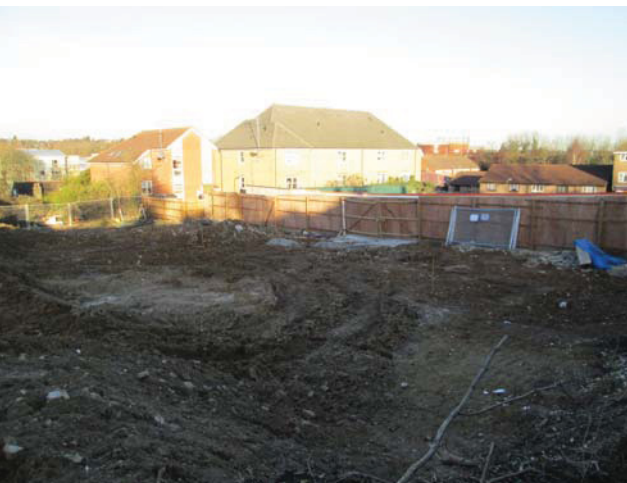
DP 17. Area 3. Looking north-west.
