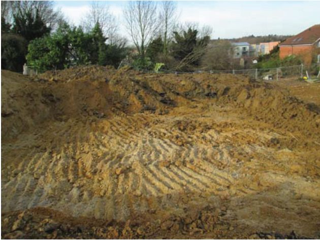
DP 19. Area 3, central part. Looking west.
