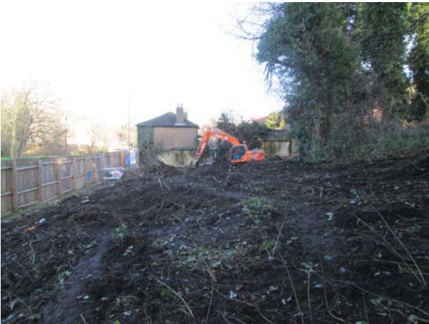
DP 1. Area 1 before commencing the groundworks. Looking north.
