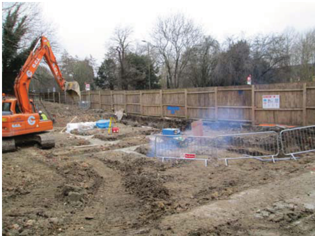
DP 11. Area 1 during construction of the foundations. Looking south-west.
