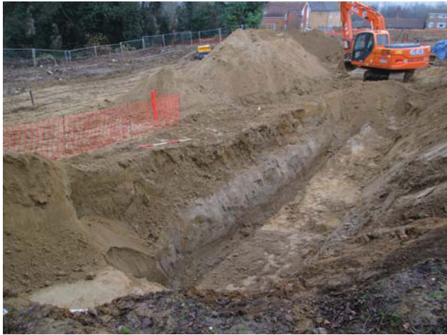
DP 21. Area 4, excavations for a new soakway. Looking north-north-west.
