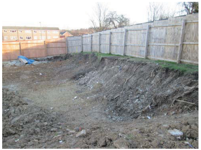
DP 18. Area 3, eastern part. Looking north.
