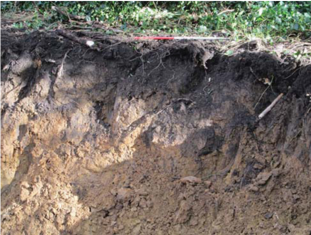
DP 3. Area 1. Excavations for a new soakway, sample section 1. Looking east.
