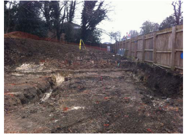
DP 4. Area 1. Reinstated ground and foundation trenches. Looking south.
