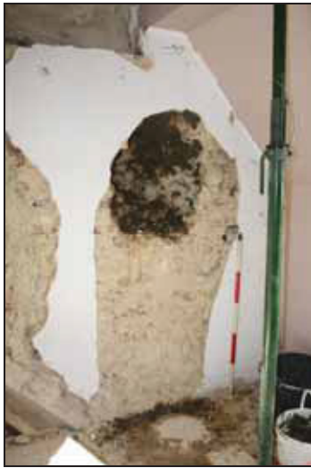
DP 105 View of the south side of the chancel arch during the piercing of the southern doorway, taken from the north-west
