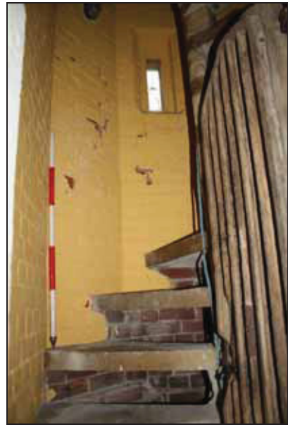
DP 52 View of staircase on the south side of Room GF04, taken from the north
