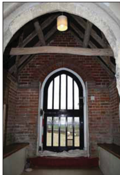
DP 54 South porch Room GF05, taken from the north
