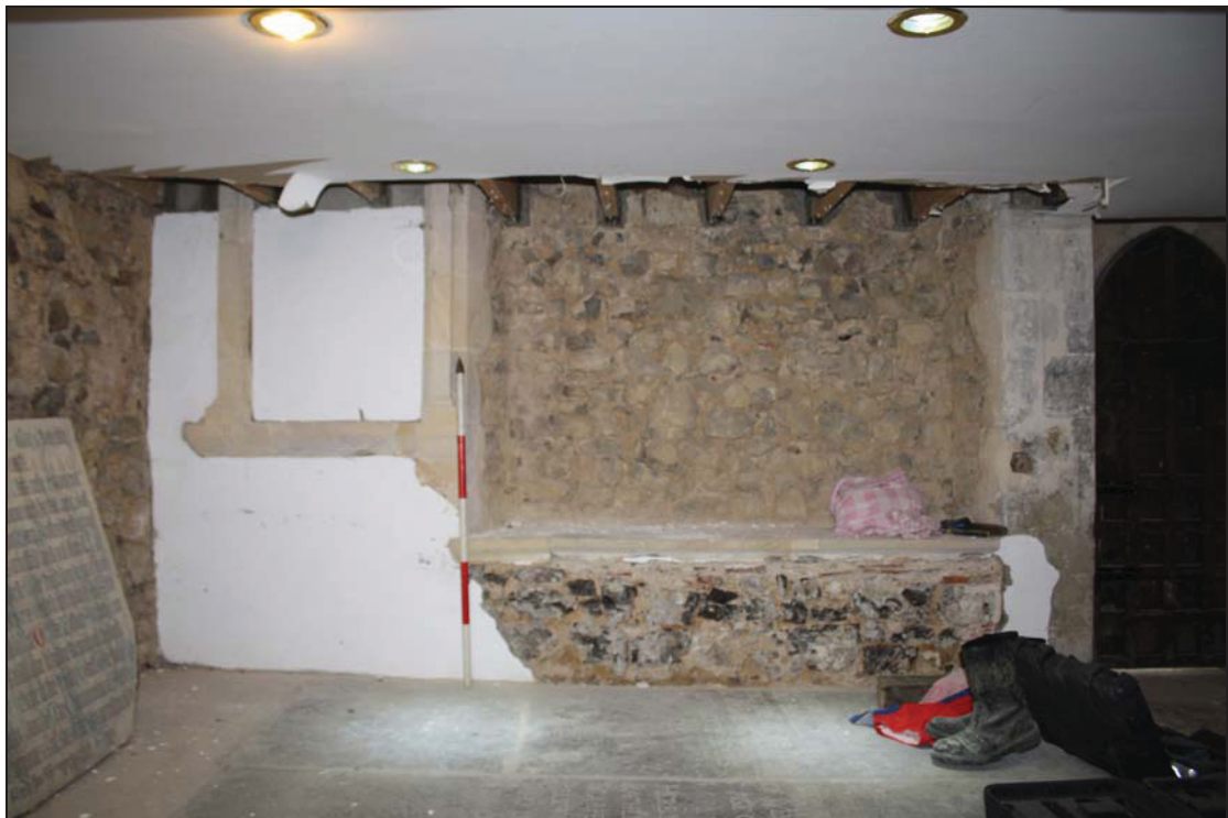
Plate 6 South wall of Room GF01 (chancel), taken from the north (DP 25)
