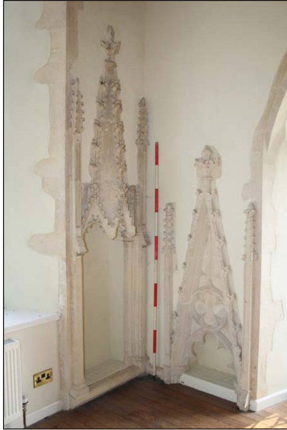
Plate 7 Hoods of image niche and piscina in the south-east corner of Room FF01, taken from the north-west (DP 46)
