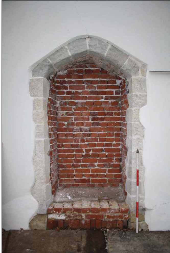
Plate 3 Blocked doorway on the north side of the chancel, taken from north (DP 12)
