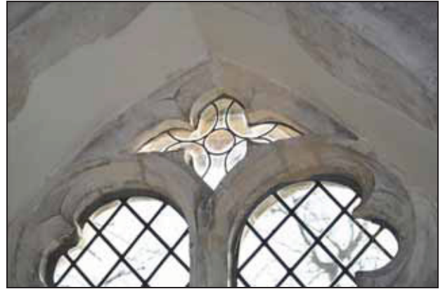
DP 50 Detail of window on the south side of Room FF01 showing early glass, taken from the north
