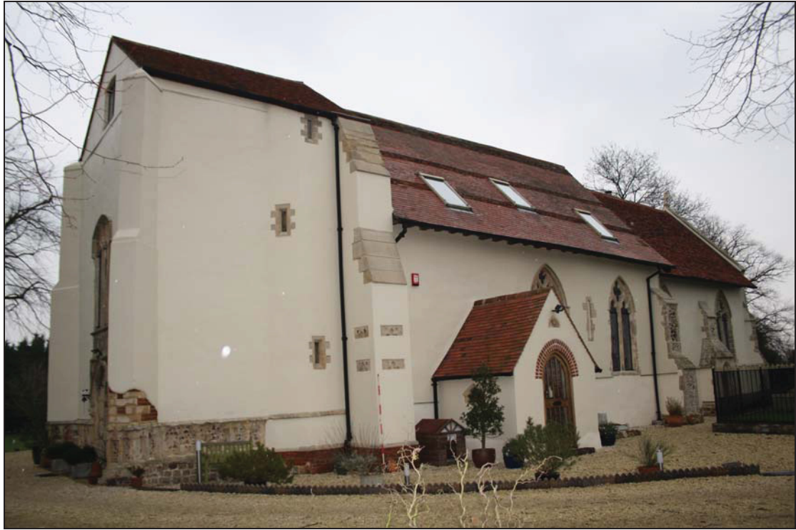
Plate 1 South elevation, taken from the south-west (DP 06)
