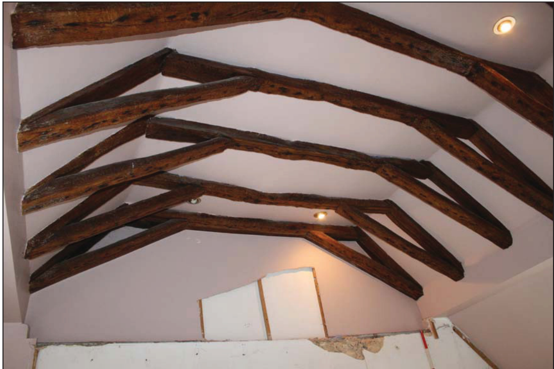
Plate 9 Roof structure in Room SF01, taken from the east (DP 36)
