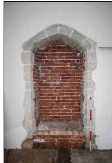
DP 12 Blocked doorway on the north side of the chancel, taken from north
