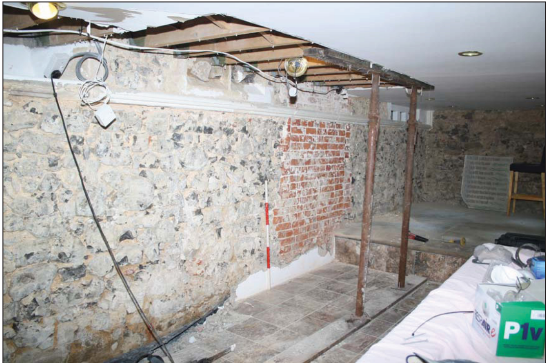
Plate 5 North wall of Room GF01 (chancel), taken from south-west (DP 15)
