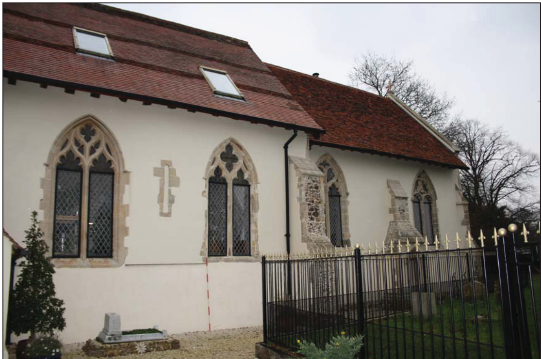
Plate 2 South elevation of the nave and chancel, taken from the south-west (DP 08)
