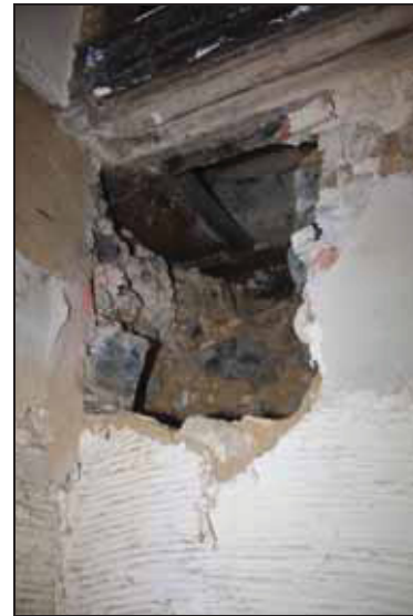
DP 118 Floor socket 9 on the south side of the nave during the planned works, taken from the north
