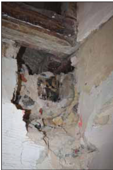
DP 119 Floor socket 5 on the north side of the nave during the planned works, taken from the south
