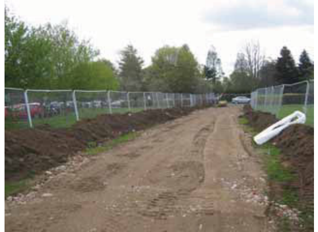
DP 2 Temporary access road, taken from the north-west
