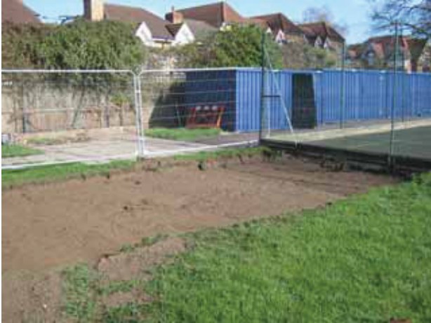
DP 1 Topsoil strip, taken from the south
