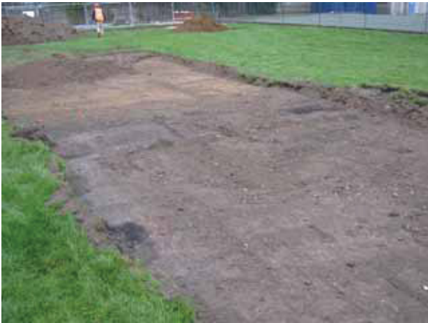
DP 3 Topsoil stripped for the site compound, taken from the south-east
