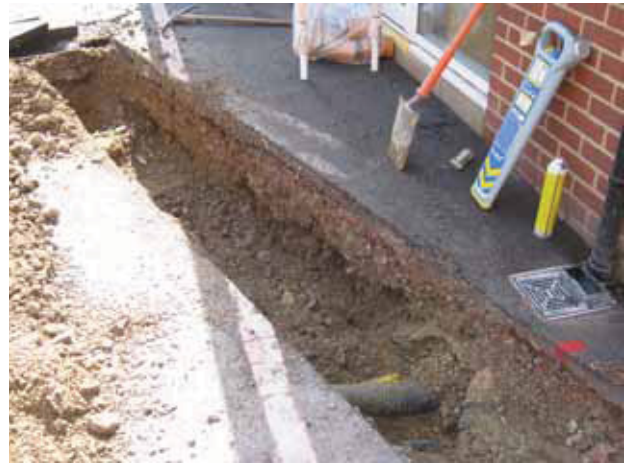
DP 4 Service trench monitored during first visit, taken from the south-east
