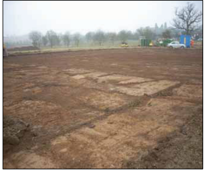
6 General view of topsoil strip of car park area looking south-east
