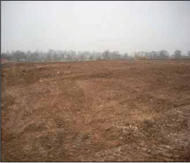
5 General view of topsoil strip of playing fields area looking south
