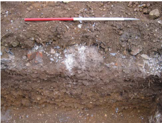
DP 5. Foundation trench, NE part. Sample section. View SW.
