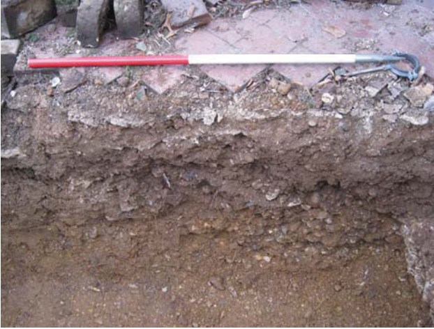
DP 7. Foundation trench, S part. Sample section. View SW.
