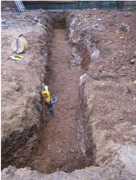
DP 3. Foundation trench, NE part. View NW.
