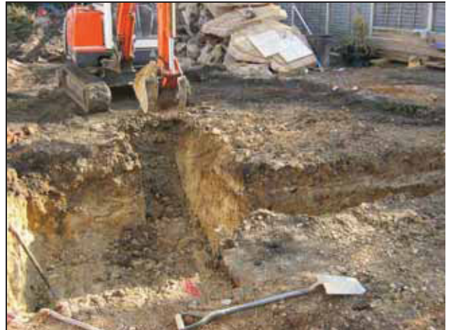
2 Mid excavation. Looking south-east.
