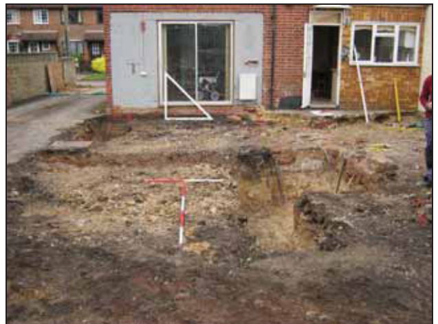
6 Post excavation. Looking north-west.
