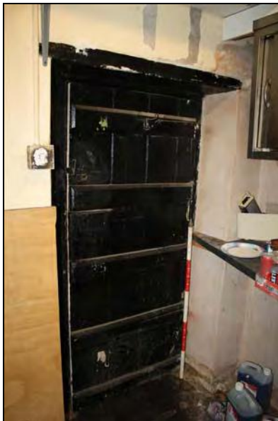
23 Rear face of door in Room GF06, taken from the south-east
