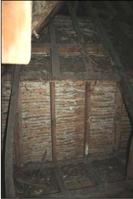
Lath and plasterwork on the north side of Room SF02 from within the adjoining roof space, taken from the north
