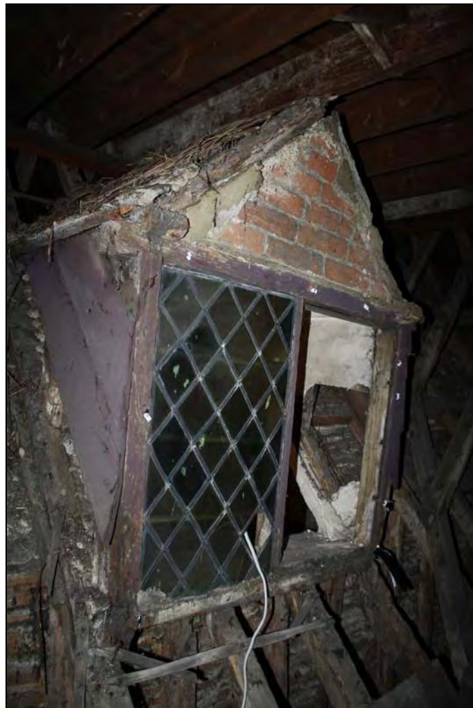
Plate 10 Original west dormer window, now entombed, taken from the north-east (51)
