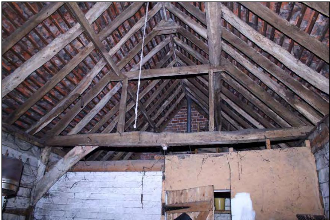
Plate 12 West truss of Room GF07 (east range), taken from the east (26)
