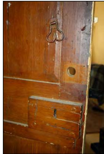
40 Drop handle and rim-lock to the original door in Room FF01, taken from the north
