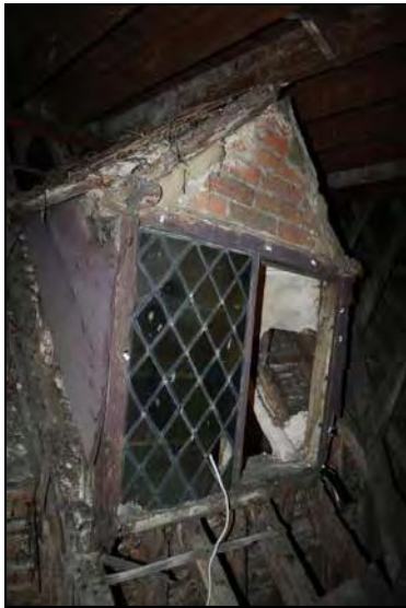
51 Original west dormer window, now entombed, taken from the north-east
