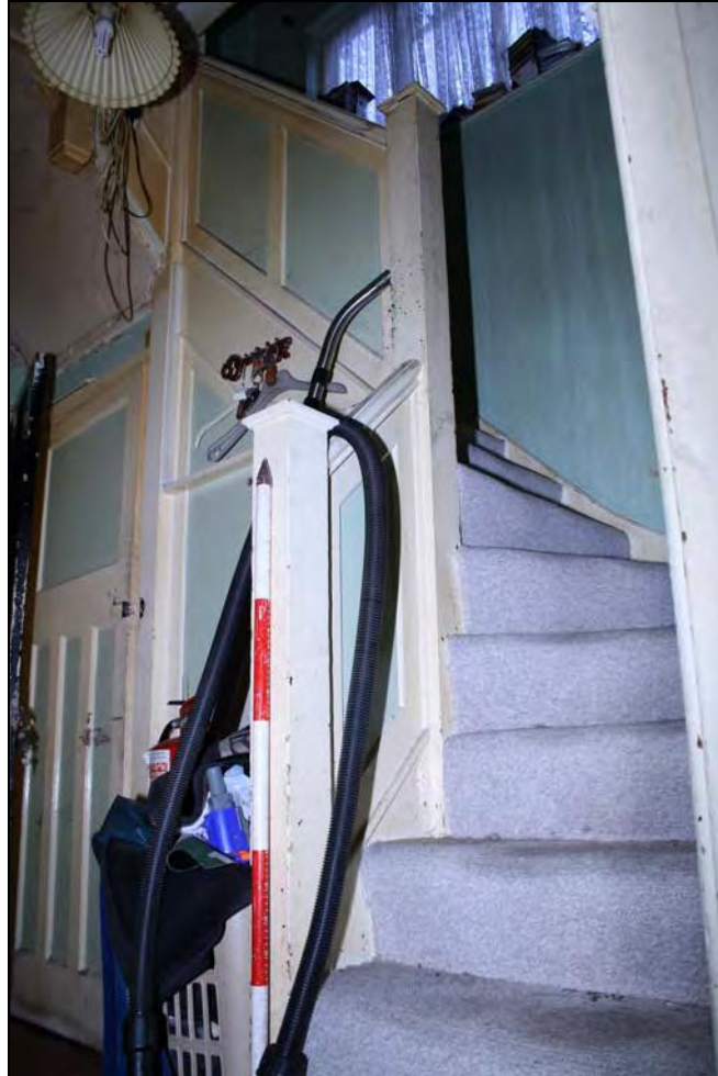
Plate 5 Staircase in Room GF04, taken from the south-east (21)
