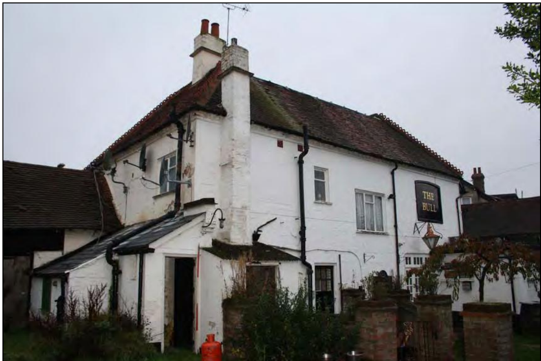
Plate 2 East and north elevation, taken from the north-east (5)
