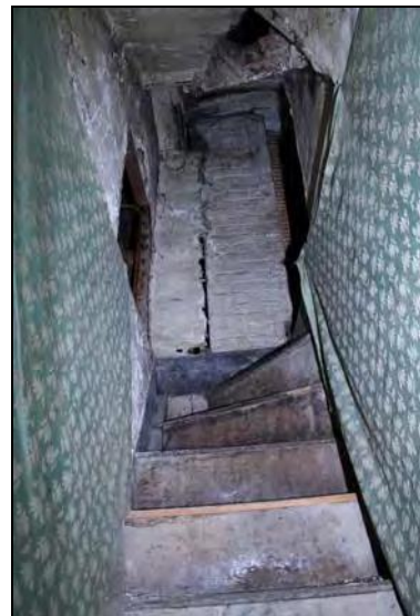
42 Staircase up to attic level, taken from the west
