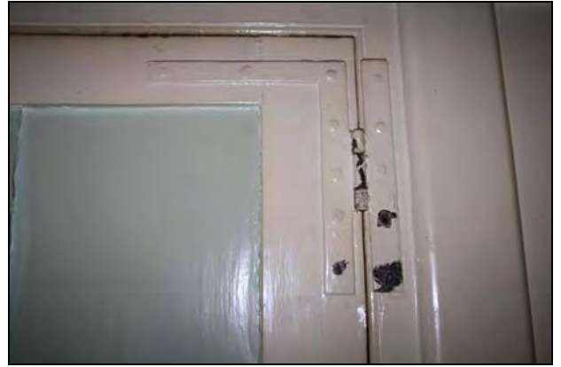
H-L hinge to the original door on the east side of Room FF01, taken from the west
