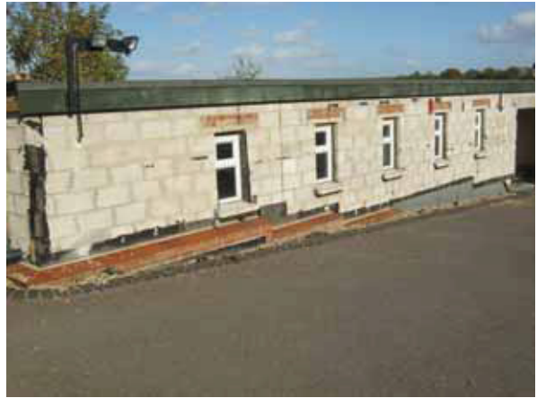
4: Outbuilding still standing on proposed location of Trench 1. Looking north-east.
