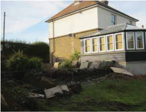
1: General view of the rear of N° 50 Green End Braughing, Herts. Looking north-west.
