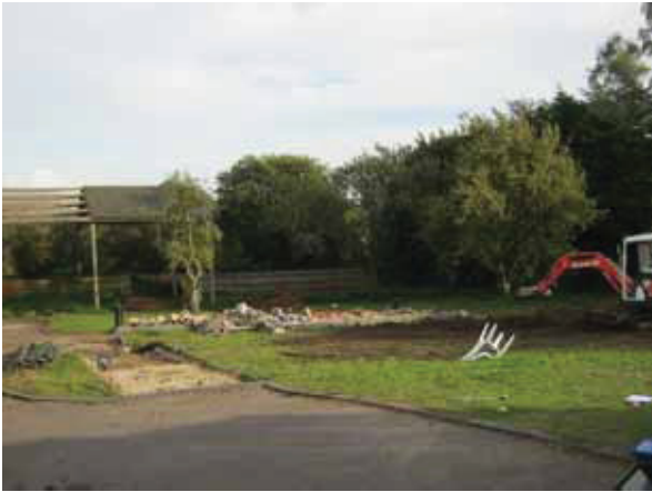
3: General view of the site. Looking east.
