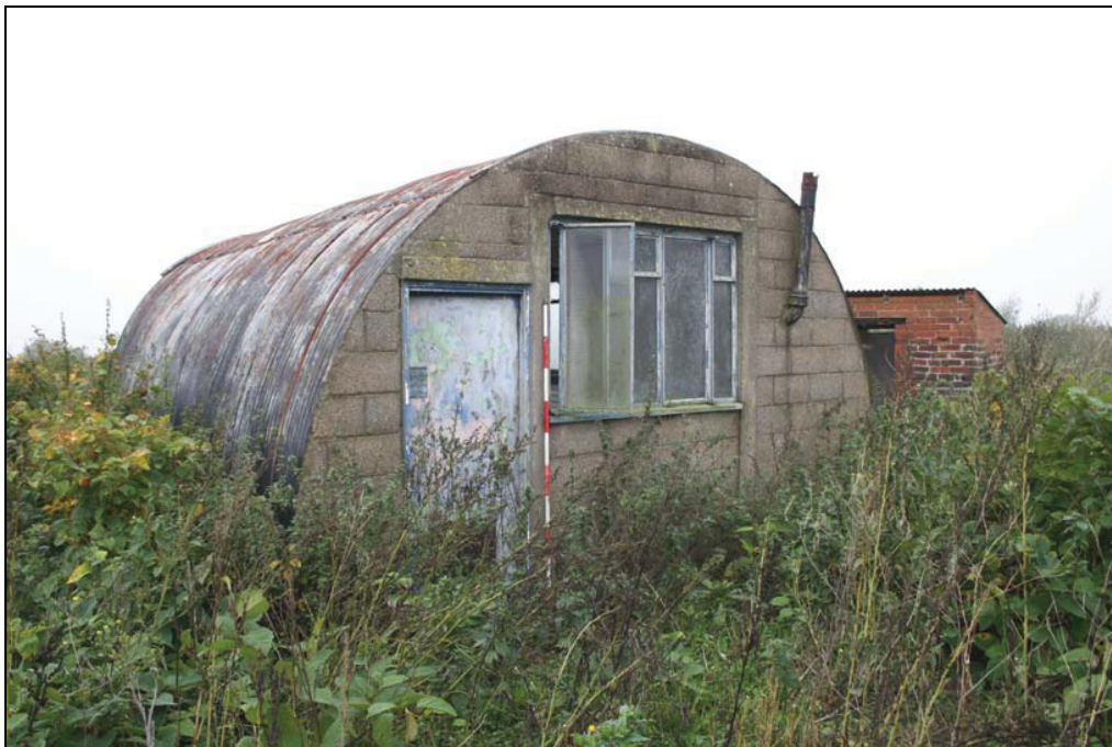
Plate 12 Nissen Hut, Building 6, taken from the north-east (DP 28)
