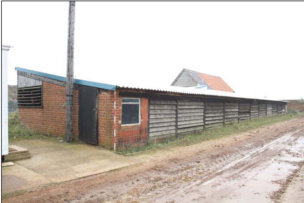
Plate 7 Drying and storage shed, Building 3, taken from the north-east (DP 11)
