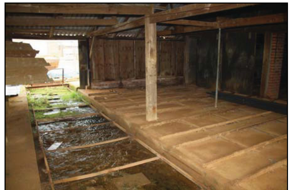
Series of trackways with a lateral track and surviving moveable trolley, north end of Building 1, taken from the north-west
