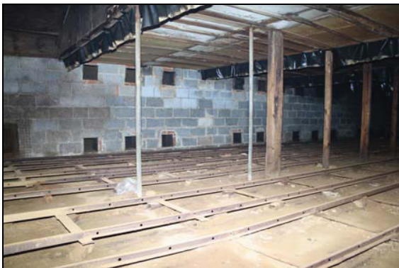
Moveable trolley and track linking internal tracks with an external track leading to the kilns, taken from the north-west
