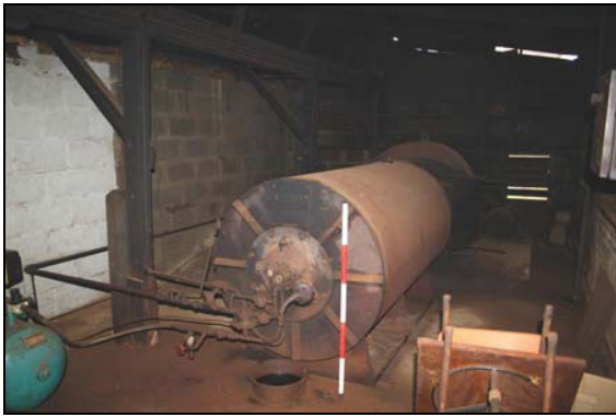
Swirlamiser oil burner housed within pent-roofed lean-to adjacent to Building 1, taken from the south-east
