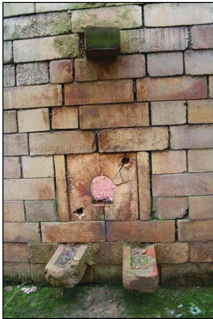
Pipe inlet into kiln, Building 2, taken from the north
