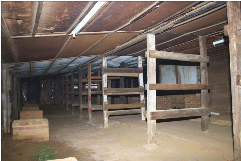
Plate 8 Partitions for shelving, interior, Building 3, taken from the south-west (DP 76)
