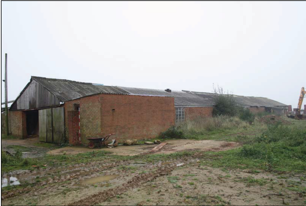
Plate 1 Main brick making building, Building 1, taken from the north-west (DP 5)
