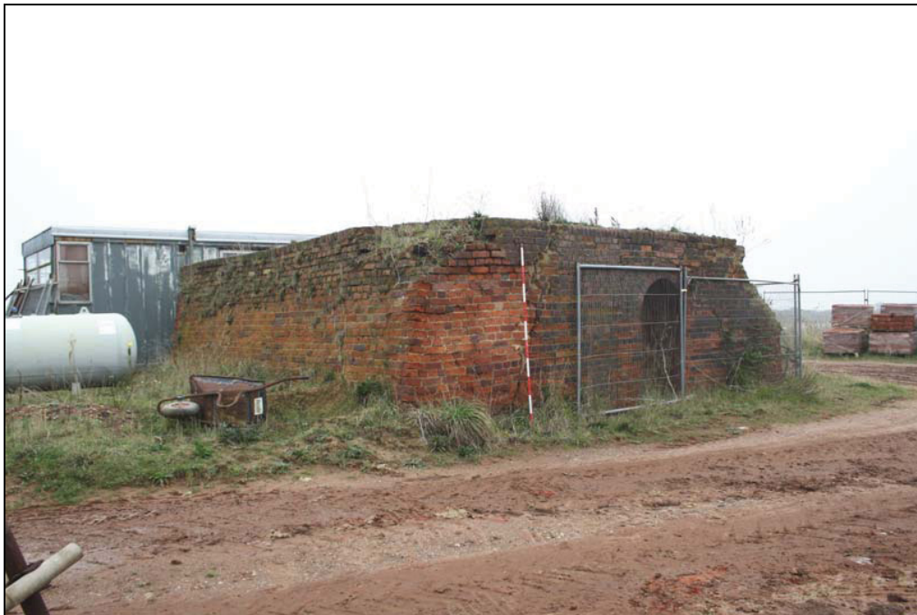
Plate 10 Early kiln, Building 4, taken from the north-west (DP 41)
