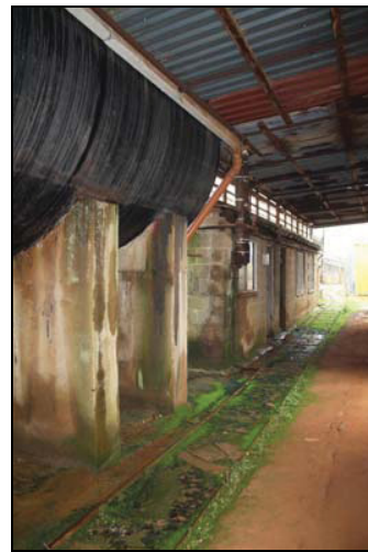
Passageway between Building 1 and kilns (Building 2) with pent roofed lean-to, oil tank and trackway, taken from the south-east
