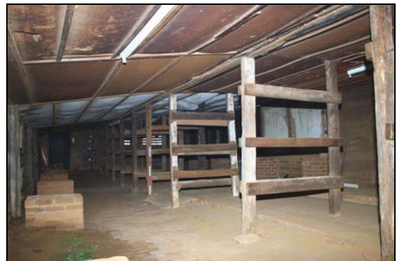
In-line tracks with lateral track and moveable trolley, interior, Building 3, taken from the north-east
