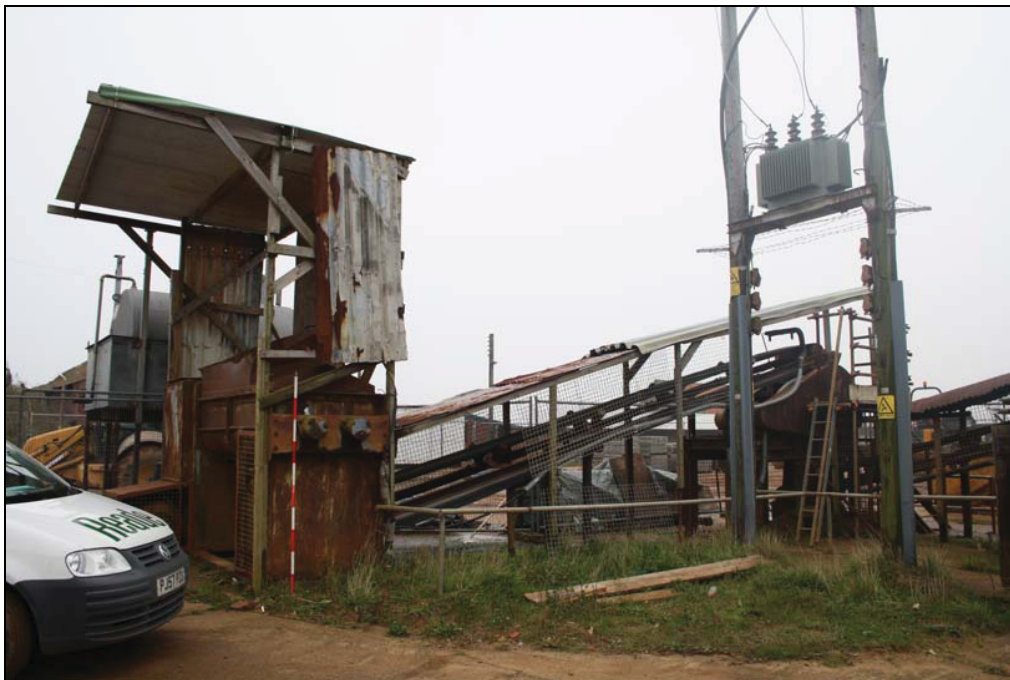
Plate 2 External machinery and conveyor belts, taken from the north-west (DP 9)
