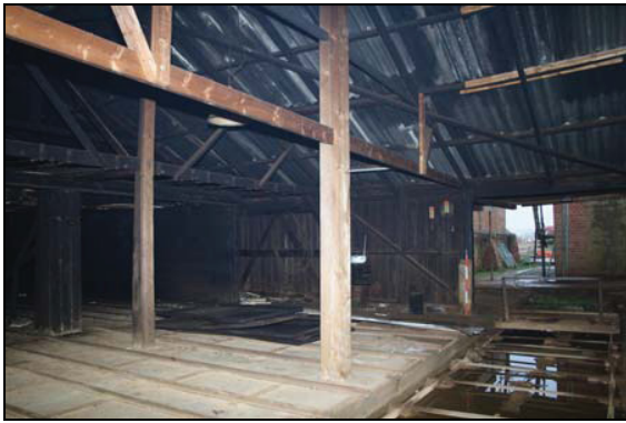
South end of Building 1 with corresponding lateral trackway and moveable trolley, taken from the south-west
