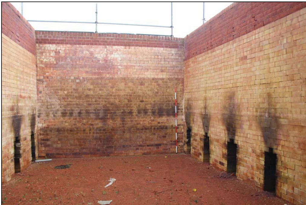
Plate 6 Kiln (Building 2), interior, taken from the north-west (DP 70)
