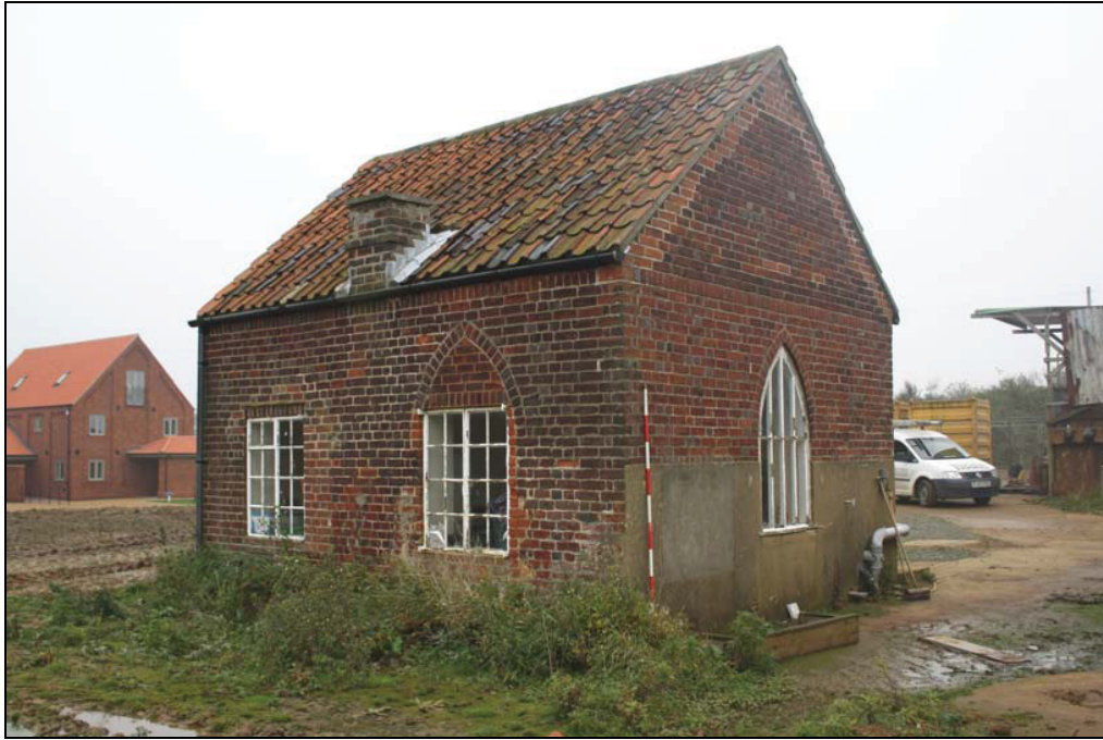
Plate 11 Building 5, south and west elevation, taken from the south-west (DP 4)
