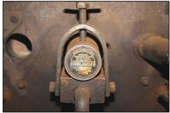
Swirlamiser oil burner housed within pent-roofed lean-to adjacent to Building 1, taken from the south-east
