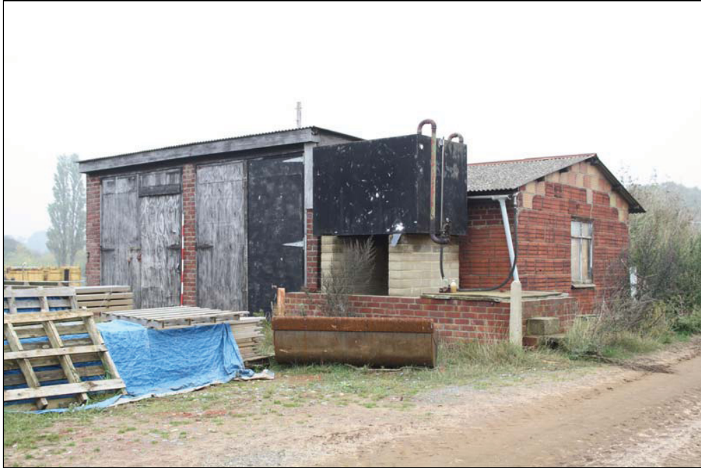
Plate 13 Storage building, Building 7, taken from the south-east (DP 35)
