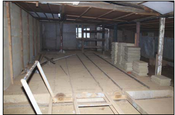
In-line tracks with lateral track and moveable trolley, interior, Building 3, taken from the north-east
