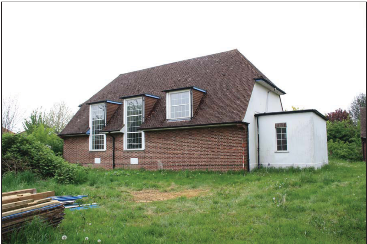
Plate 2 West elevation of the church, taken from the south-west (DP 02)
