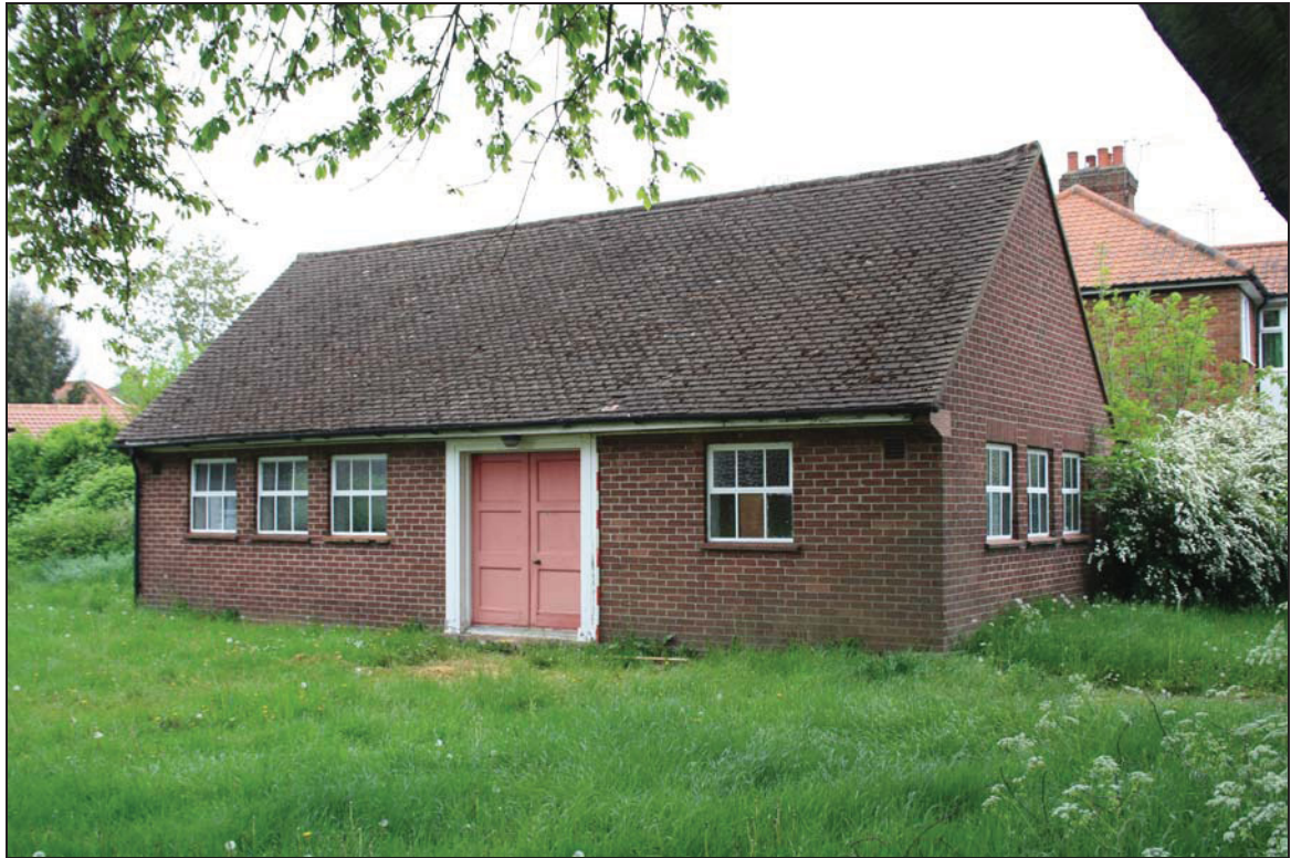
Plate 5 West elevation of Building 2, taken from the south-west (DP 8)
