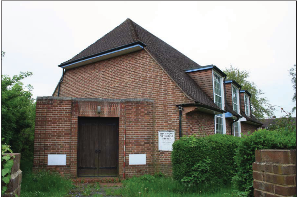
Plate 1 North elevation of the church, taken from the north-west (DP 1)
