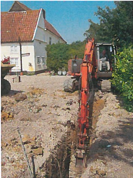
Excavation of footing trench.. Looking west.
