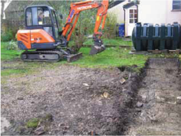
1 Topsoil stripping looking south-west
