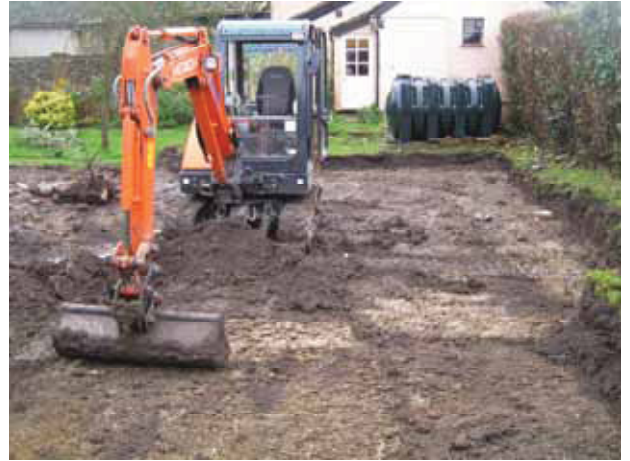
2 Area after stripping looking south-west
