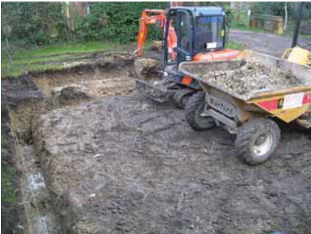
3 Excavating the footings looking north
