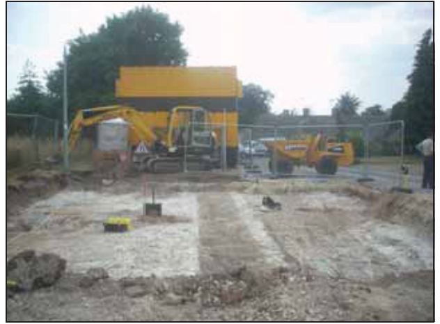
2 Site after topsoil stripping ( July 2013 )
