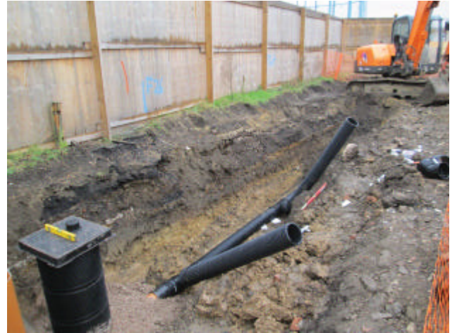
DP 4. Drainage trench. Looking south-south-west.
