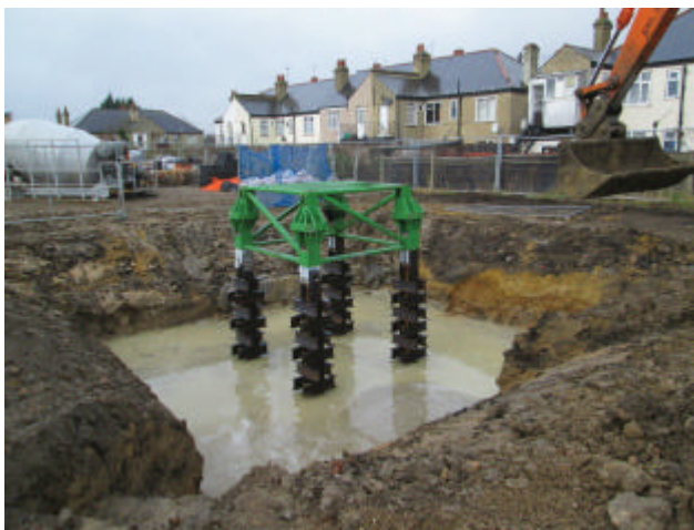
DP 9. Excavation for a crane base. Looking west.
