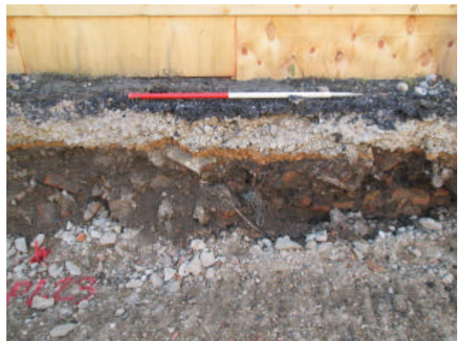
DP 12. Ground reduction, sample section 5. Looking south-east.
