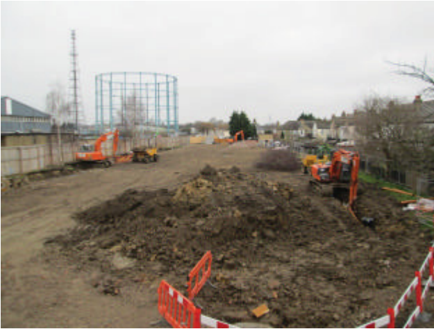
DP 1. The site. Looking south-west.
