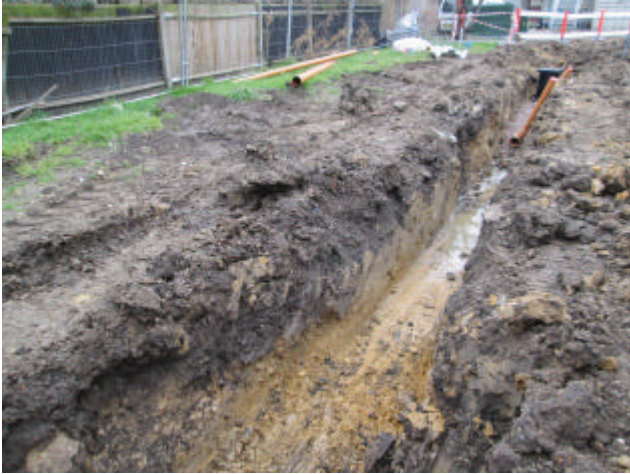
DP 7. Drainage trench in north-eastern part of the site. Looking north-east.
