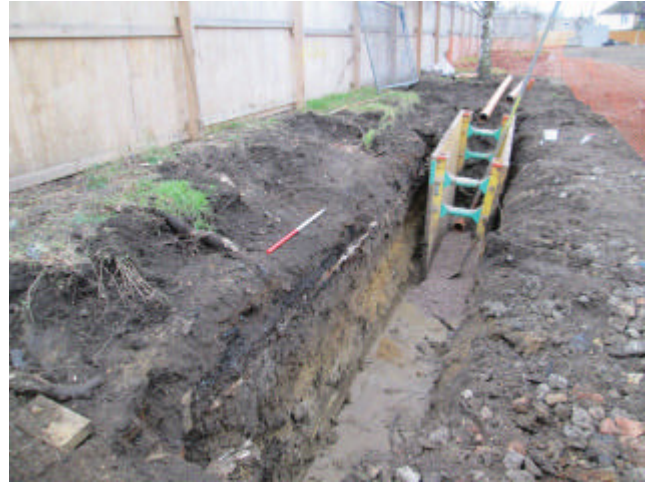
DP 2. Drainage trench along southern side of the site. Looking south-west.
