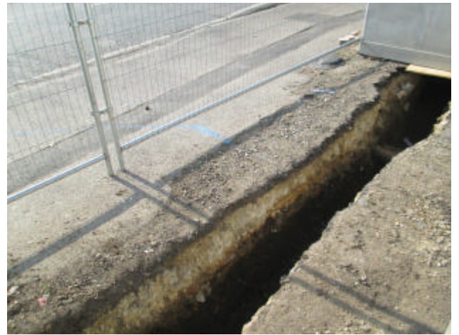
DP 6. Drainage trench, south-western section. Looking south-south-west.
