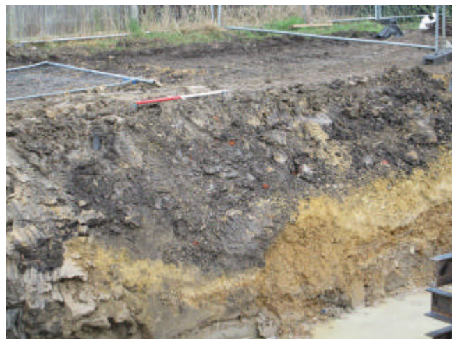
DP 10. Crane base, northern side. Sample section 4. Looking north.
