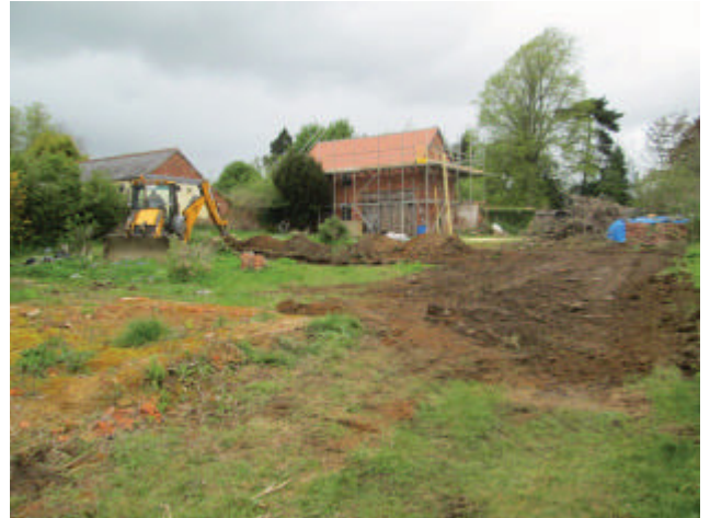
DP 2. The site. Looking north-west.
