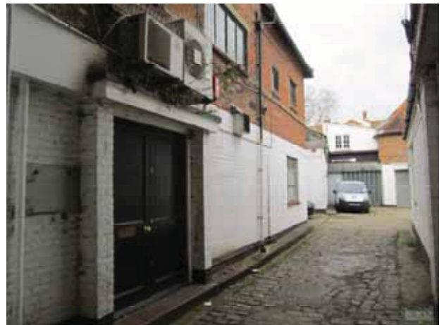
4 View NE along narrow yard leading to rear of site
