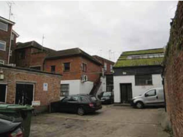
9 View W across yard to the buildings at the rear of the site
