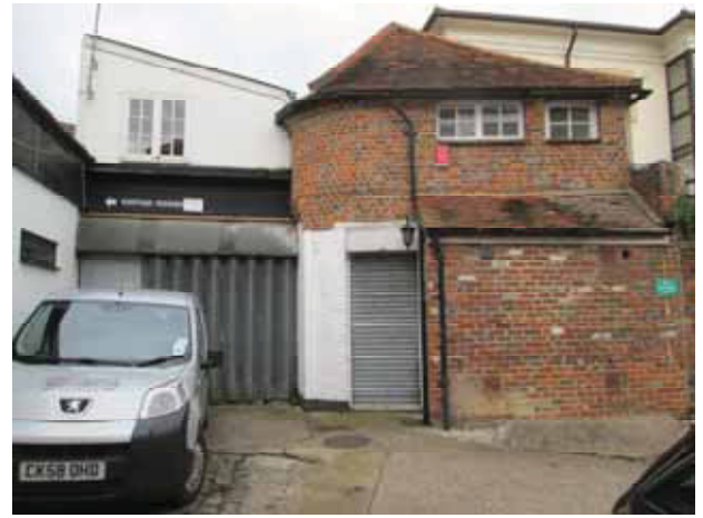
8 View E of 'corner' building adjoining the light industrial unit to the rear of the site
