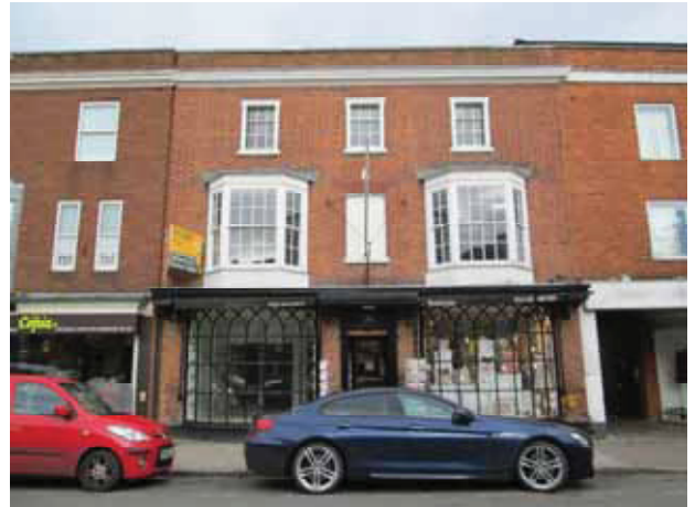
2 View E of building façade of site
