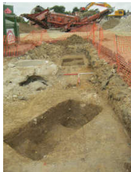
6 Trench 6 post-excitation. Looking west.
