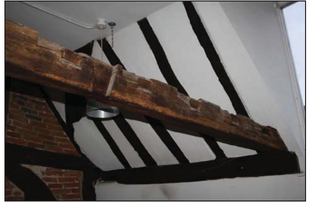
Former wall-plate redeployed as a binding joist in Room FF01, Range 1, taken from the south
