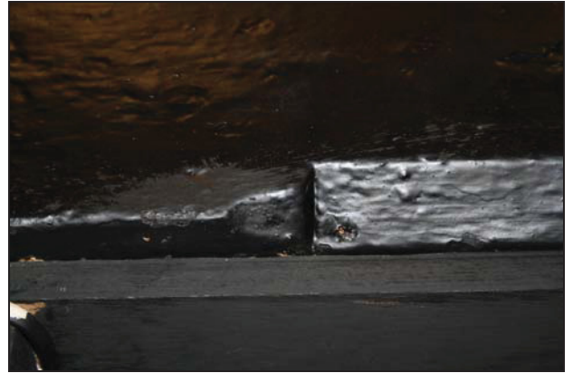
Lamb's tongue chamfer stop on the fireplace lintel now facing into Range 2, taken from the east
