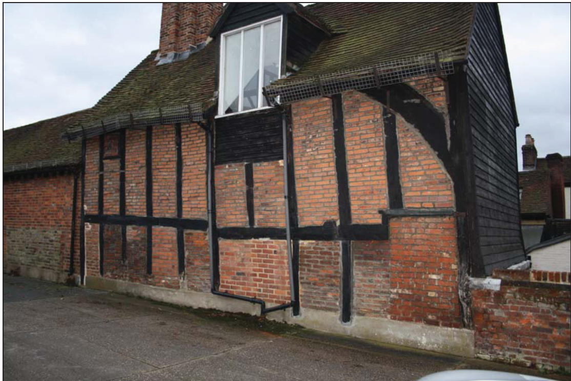
Plate 2 Northern elevation of Range 1, taken from the north (DP 7)
