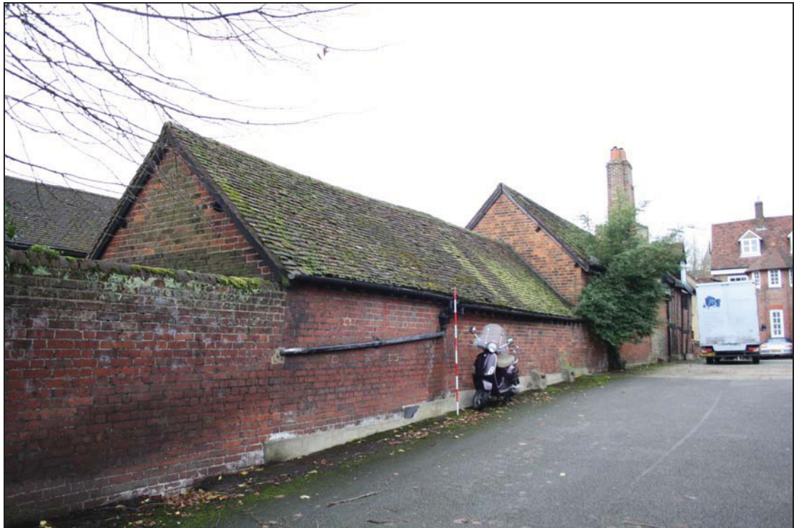
Plate 7 Northern elevations of Range 2-4, taken from the east (DP 8)
