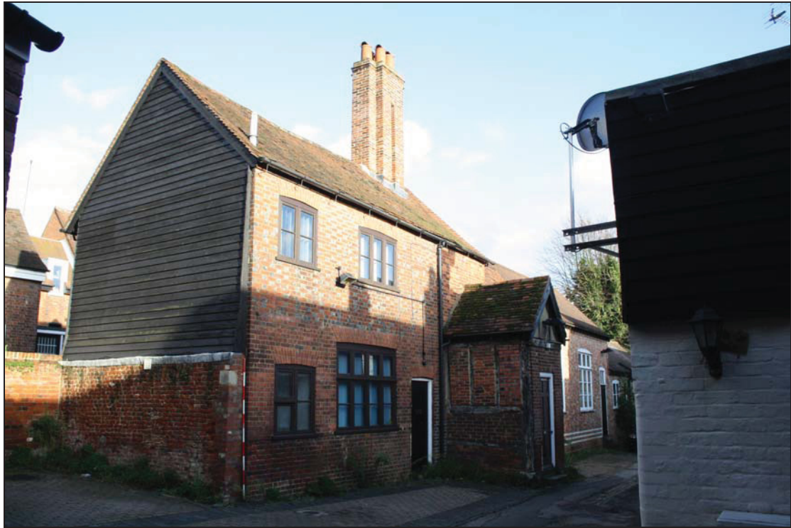
Plate 1 South side of Range 1, taken from the west (DP 1)
