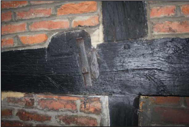
Possible internal binding joist notched over the northern mid-rail of the west bay, Range 1, taken from the north
