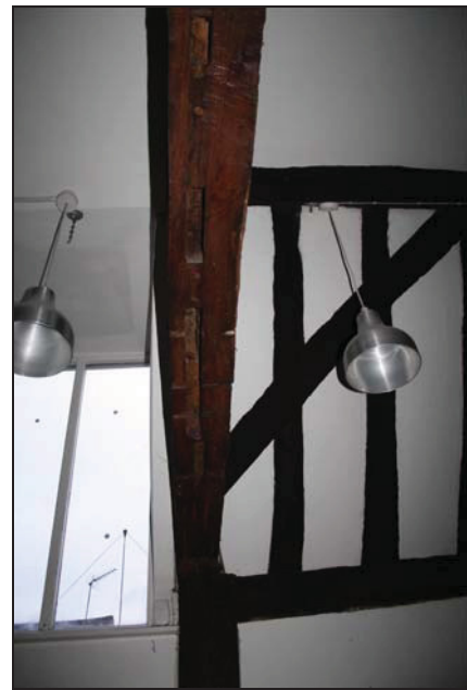
Soffit of the central tie-beam in Room FF01 showing redundant brace mortice and empty stud mortices, Range 1, taken from the south
