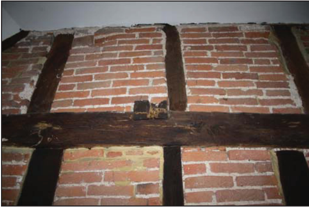
Upper section of the west wall of Room FF01 showing possible truncated bridging joist, Range 1, taken from the east
