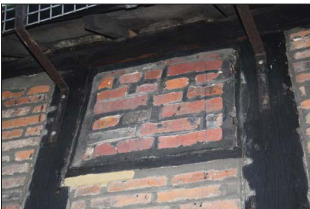
Detail of the east light of the former tripartite window on the north side of the east bay, Range 1, taken from the north
