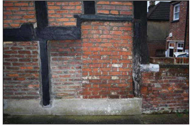
Inserted doorway on the northern side of Range 1, itself later blocked, taken from the north-east
