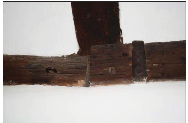
Soffit of the central tie-beam in Room FF01 showing redundant brace mortice and empty stud mortices, Range 1, taken from the south
