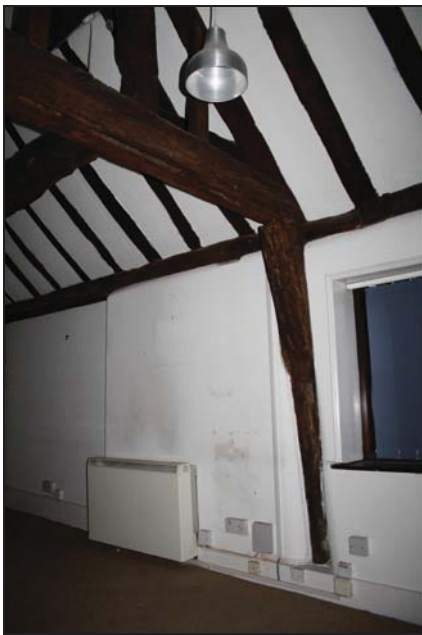
Upper section of the west wall of Room FF01 showing possible truncated bridging joist, Range 1, taken from the east
