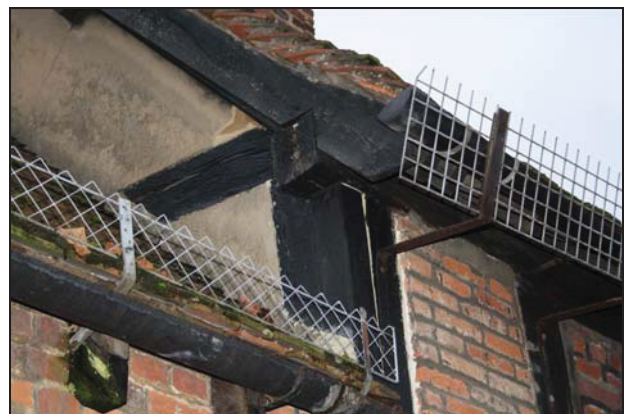
North-east corner of Range 1 showing unweathered wall-plate, taken from the north-east
