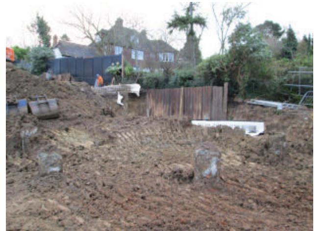
DP 12. South-western part of the excavation area. Looking south-east.
