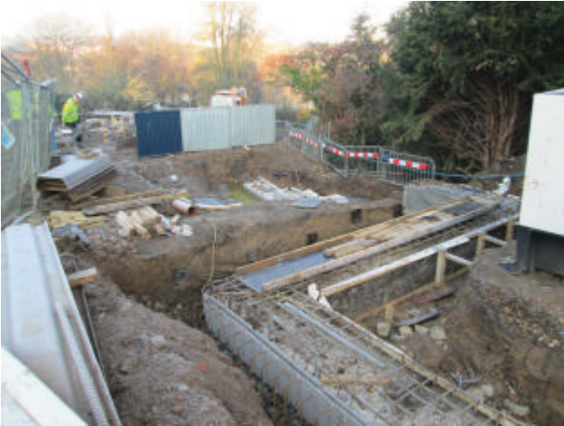
DP 3. Foundations in north-western part of the site. Looking west-north-west.
