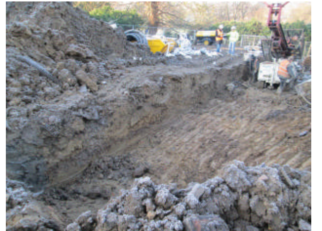
DP 10. Ground reduction in north-western part of the excavation. Looking south-west.
