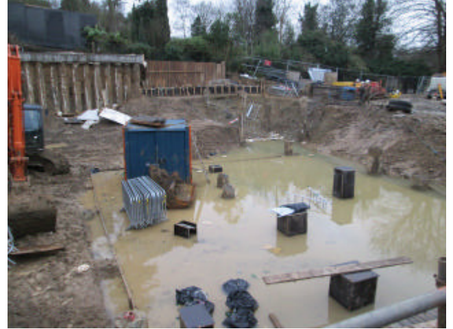
DP 20. Central/western part of the site. Looking south-south-west.
