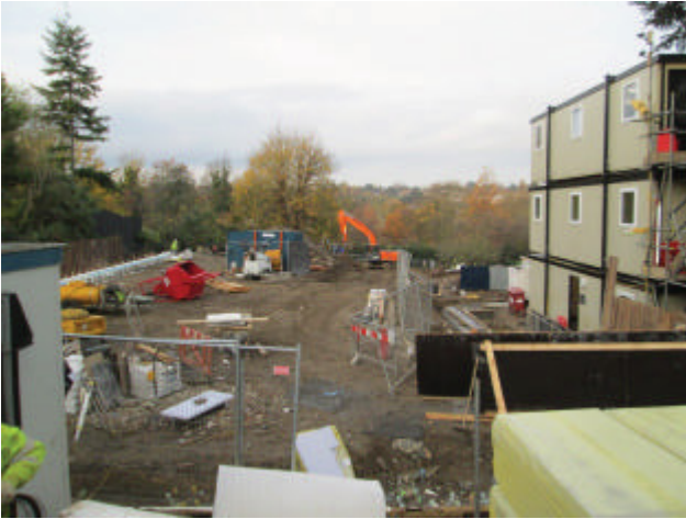
DP 1. The site in early stage of works. Looking west.
