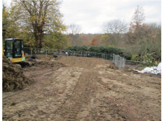
DP 2. Southern part of the site. Looking west.
