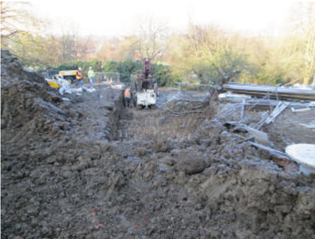
DP 9. North-western part of the excavation area. Looking west.
