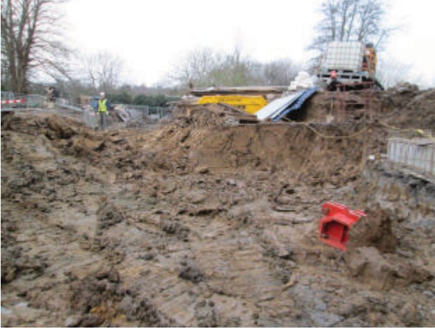
DP 13. Central part of the site during ground reduction. Looking west.
