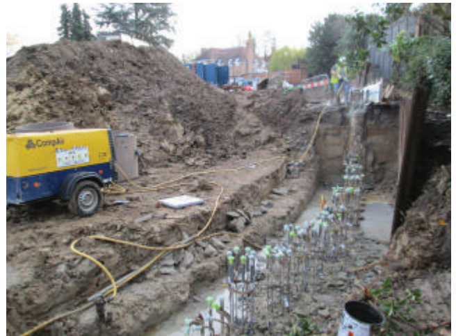
DP 6. Southern side of the excavation area, south-west part. Looking east.
