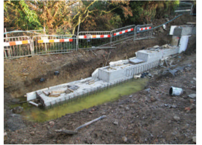
DP 4. Northern side of the excavation area, central part. Looking north-east.
