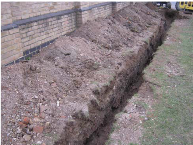
DP 3. Eastern part of the trench. Looking east.
