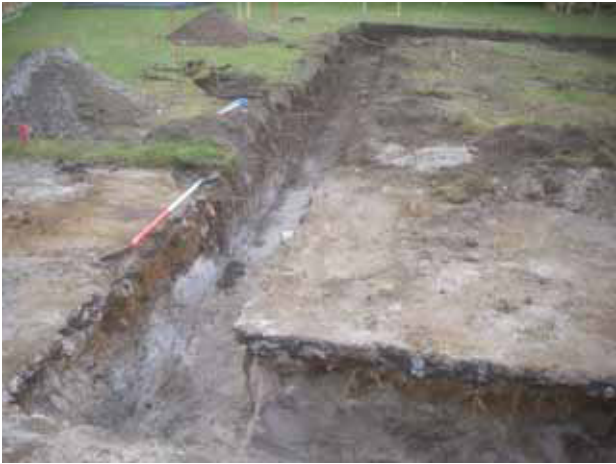
1 General shot of site looking north
