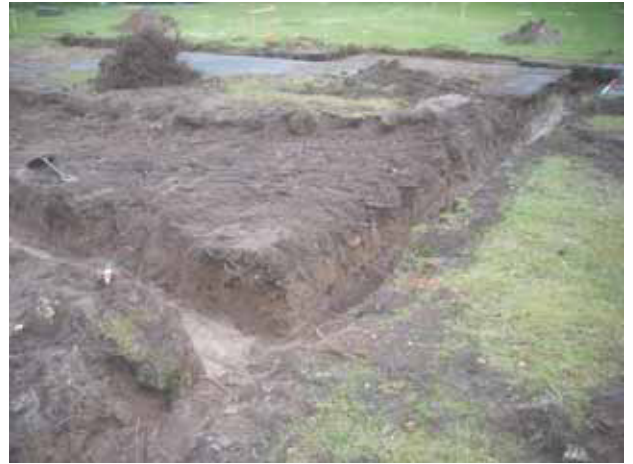
2 General shot of site looking north
