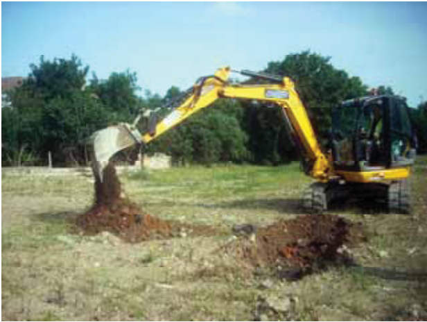
1 Test pit 1 being excavated
