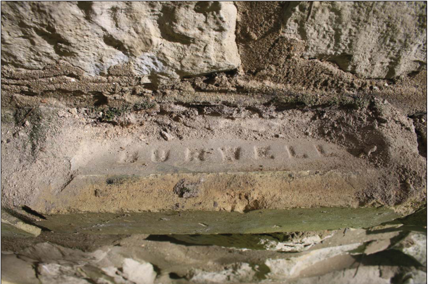
Plate 1 Burwell brick from the brick course along the top of the plinth extending around the barn, taken from the west
