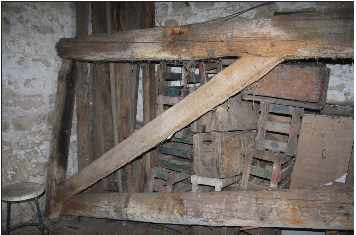
Plate 26 End of an ex-situ truss showing the earlier roof construction including tie-beam, post and brace, taken from the west
