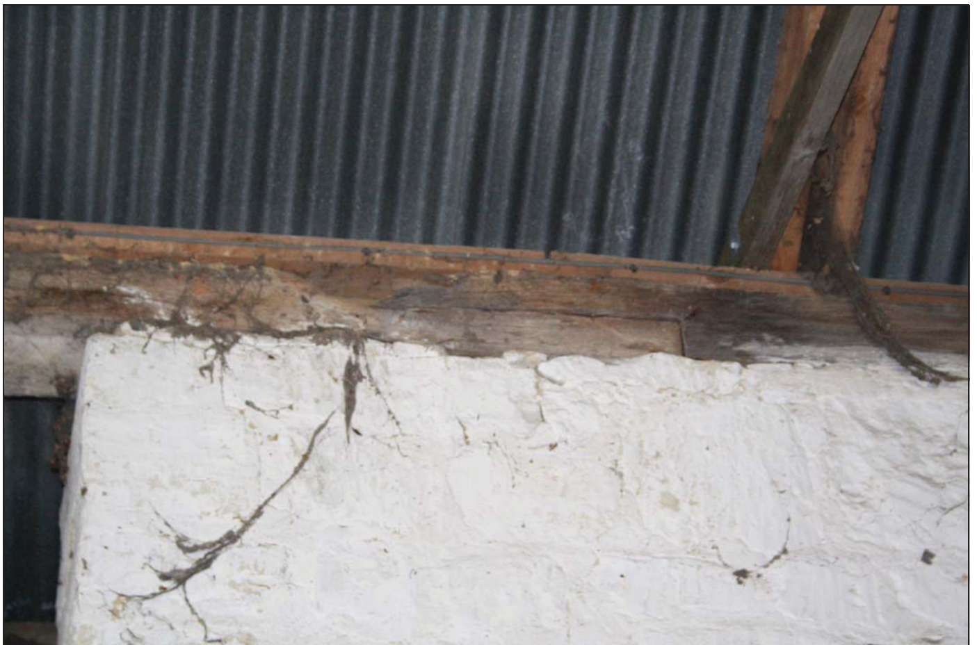
Plate 24 Edge-halved scarf joint in the west wall-plate, taken from the east
