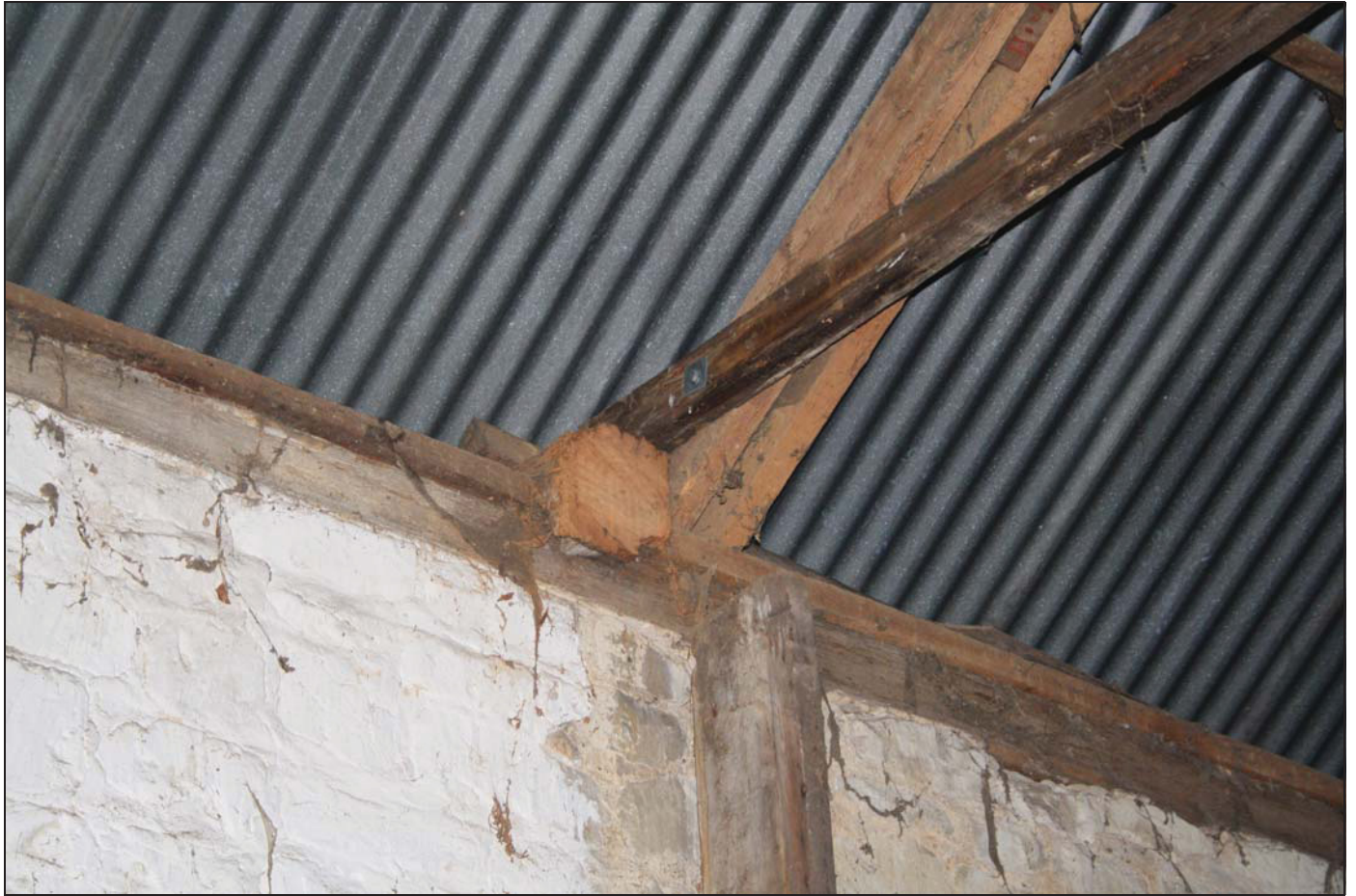
Plate 23 West side of the barn at roof level showing surviving wall plate and truncated tie-beam stump, taken from the south-east
