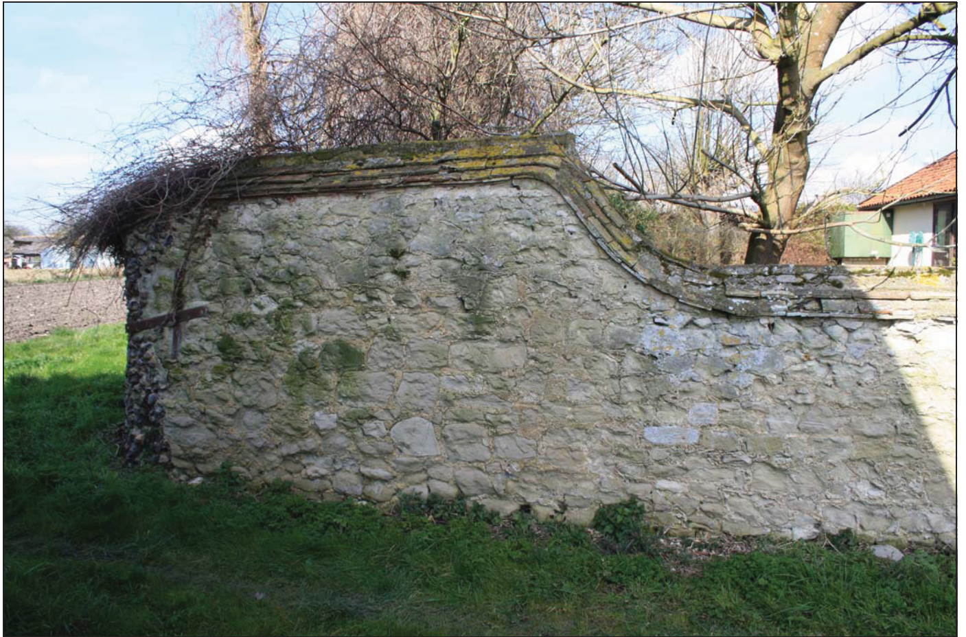
Plate 27 Retaining boundary wall of slightly varying construction to the barn enclosing The Poplars, taken from the south
