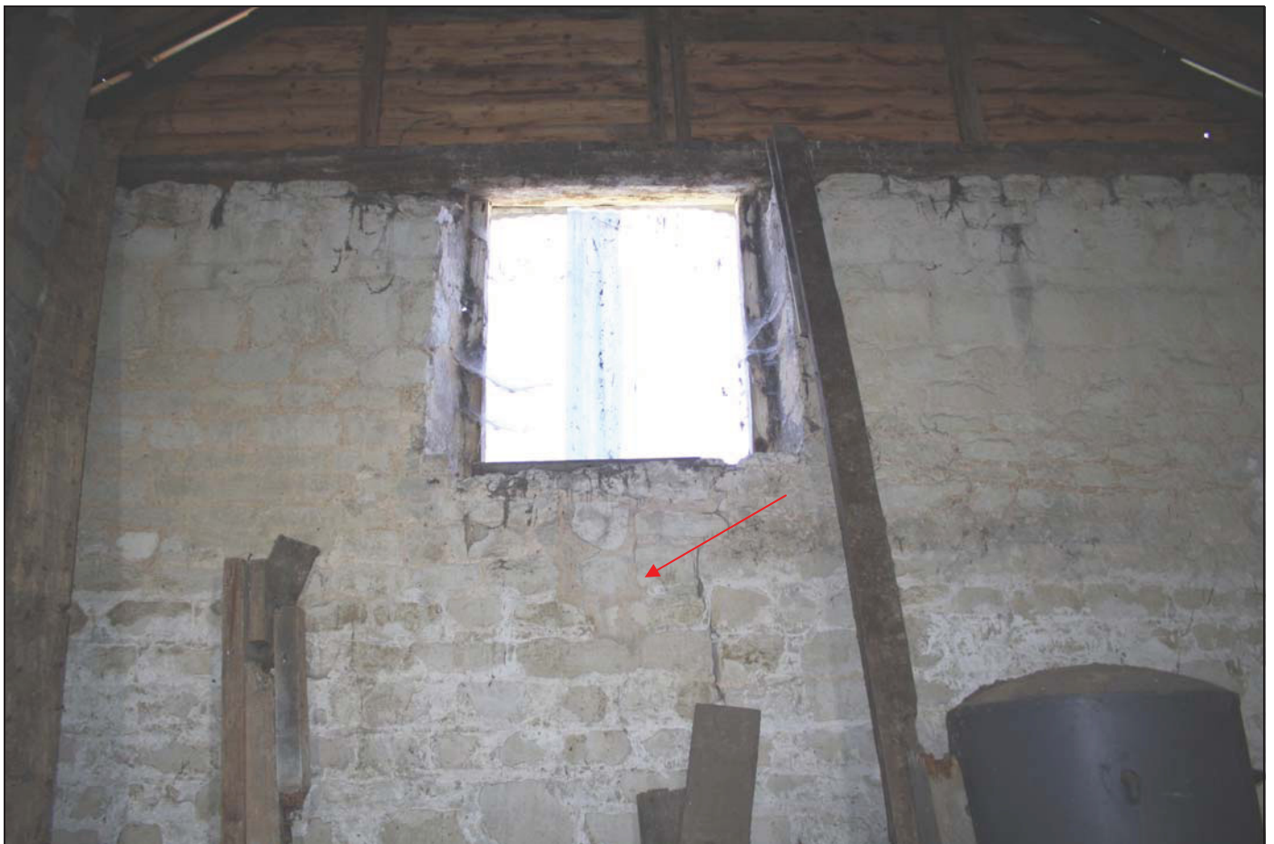
Plate 22 Inserted window at the north end of the barn with original blocked ventilation slit below (indicted), taken from the south
