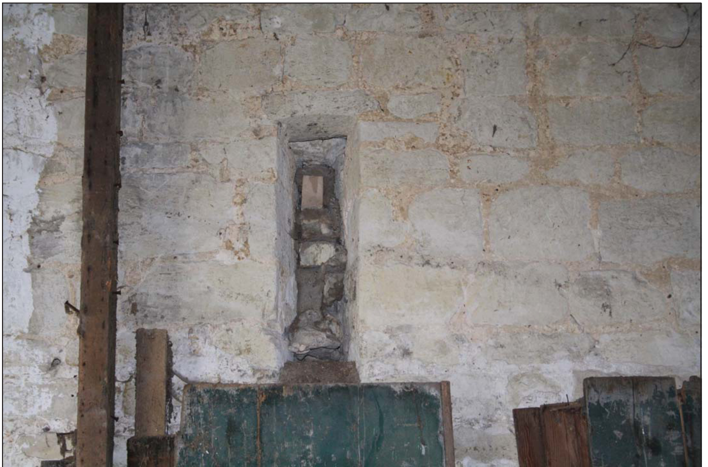
Plate 20 Blocked ventilation slit on the west side of the barn (Bay 1), taken from the east
