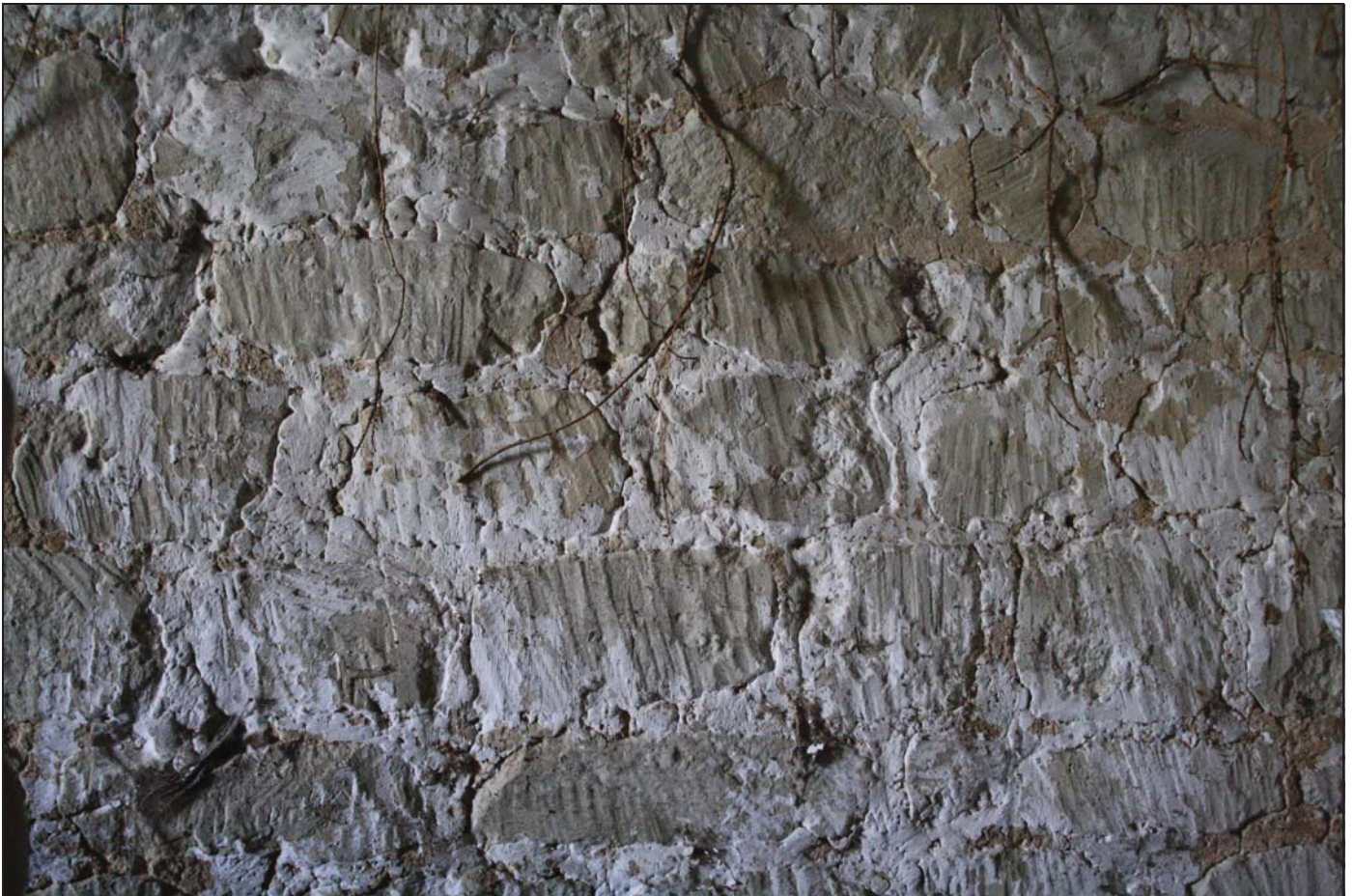
Plate 2 Example of the tooling marks on the clunch blocks on the south side of the porch, taken from the north
