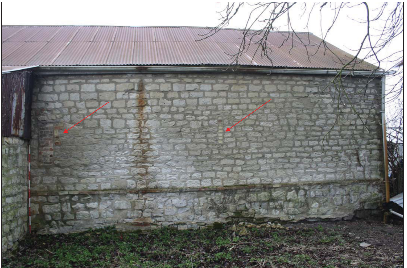
Plate 10 West elevation (south end) showing blocked ventilation slits (indicated), taken from the west
