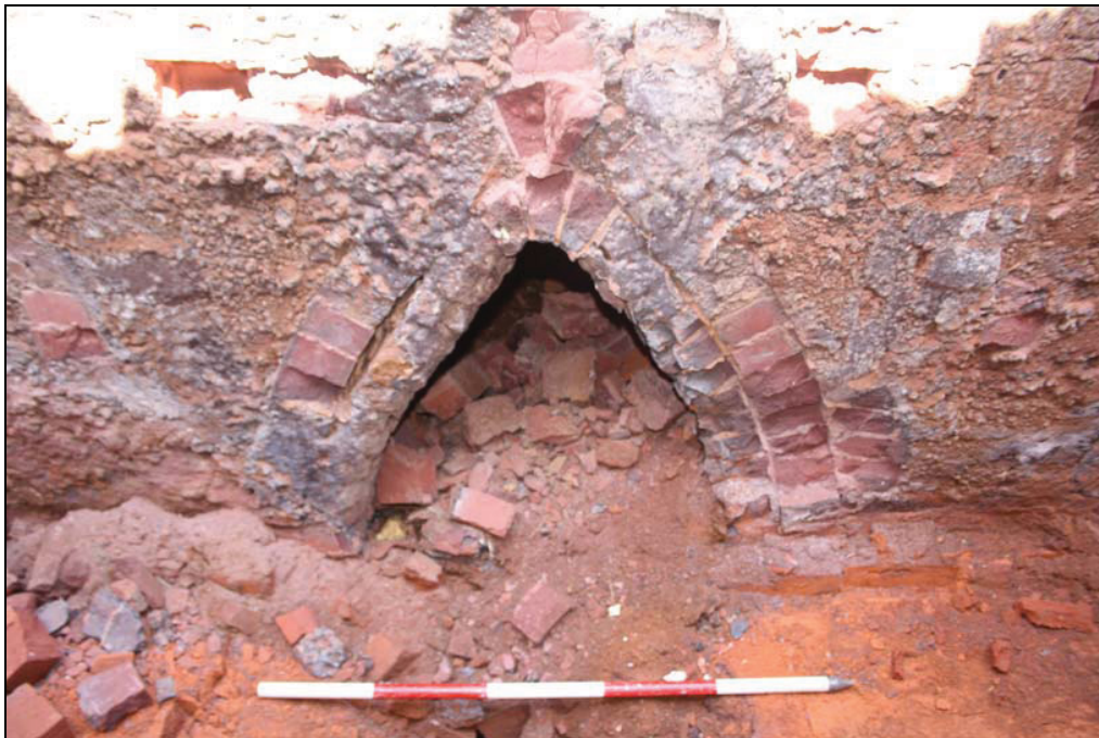
Plate 10 Detailed view of pointed arched aperture extending beneath the kiln floor, taken from the south (DP 34)
