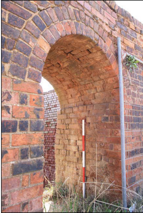
Plate 3 Central wicket, internal construction, western elevation, taken from the north-west (DP 13)
