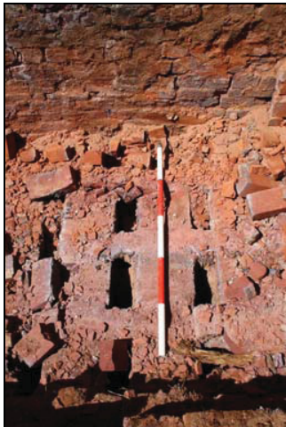
Large apertures within the brickwork make-up of the kiln floor, taken from the east
