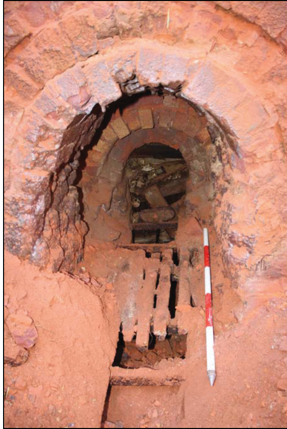
Plate 5 View through central arched aperture piercing the southern elevation with grille covered channel below, taken from the north (DP 30)
