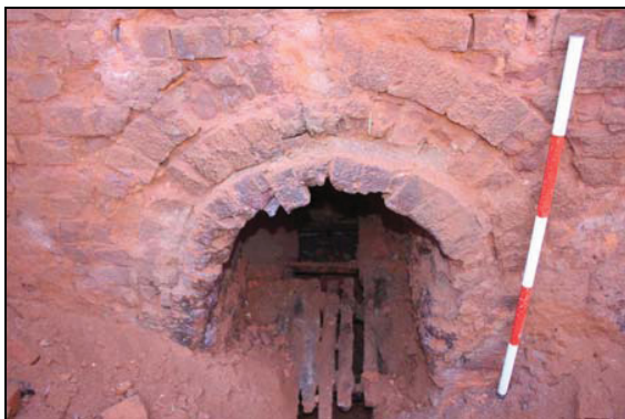
Large apertures within the brickwork make-up of the kiln floor, taken from the east
