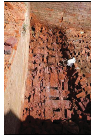
Lower level brickwork with larger apertures situated directly above fire tunnels, taken from the south
