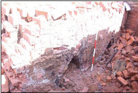
Pointed arched fire tunnels extending beneath the kiln floor, taken from the south-west
