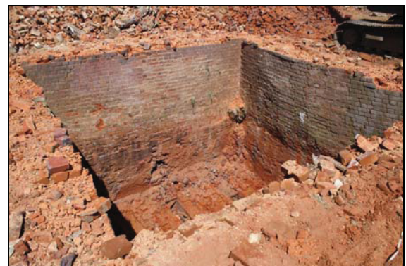
Removal of the internal floors and fire tunnels from the interior of the kiln, taken from the south-west
