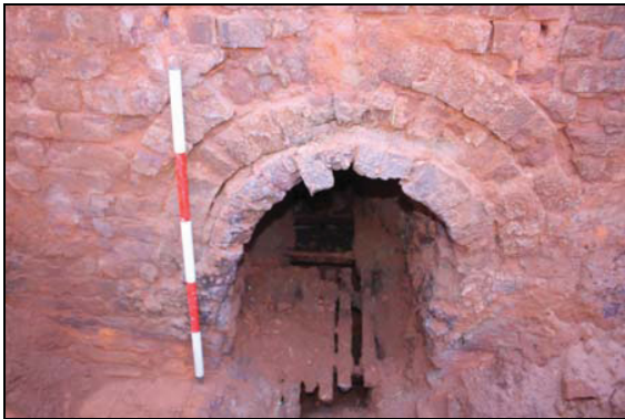
Pointed arched fire tunnels extending beneath the kiln floor, taken from the south-west
