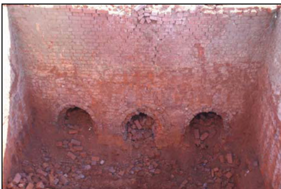
Vitrification of the brickwork within the central fire tunnel, taken from the south
