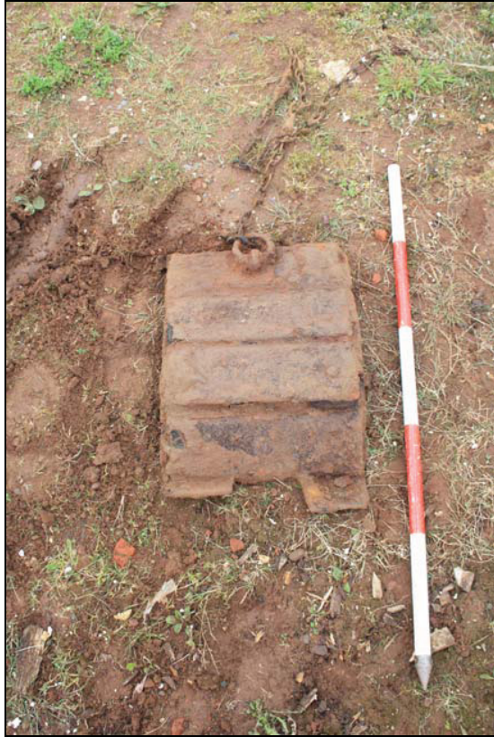
Plate 7 Heavy metal door hung on a chain used to cover one of the archways (DP 53)
