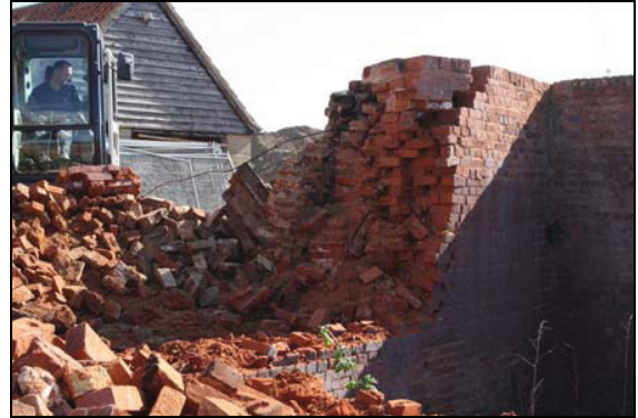
Northern elevation showing battered element as a later addition, taken from the south-west
