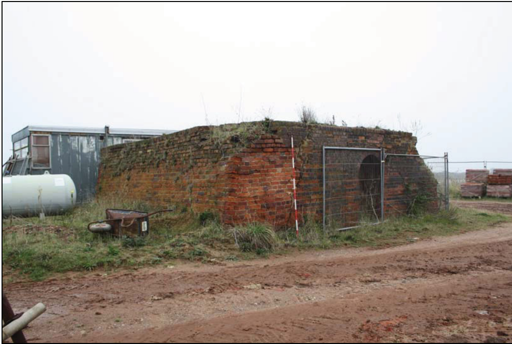
Plate 1 19 th century Suffolk kiln, taken from the north-west (DP 1)
