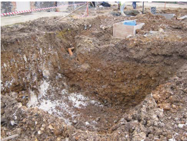
DP 11. Excavation for new soakway. Looking south-west.
