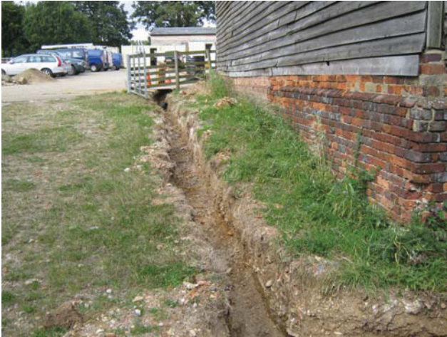
DP 1. Service trench to south-west of Maynes Cottage. Looking north-north-west.
