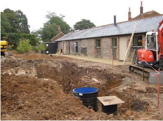
DP 7. Excavation for new biomass tank. Looking east.
