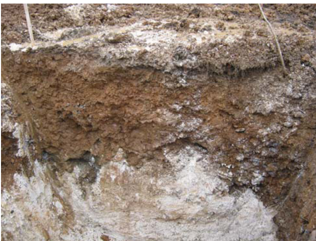
DP 9. Excavation for new biomass tank. Looking north-west.
