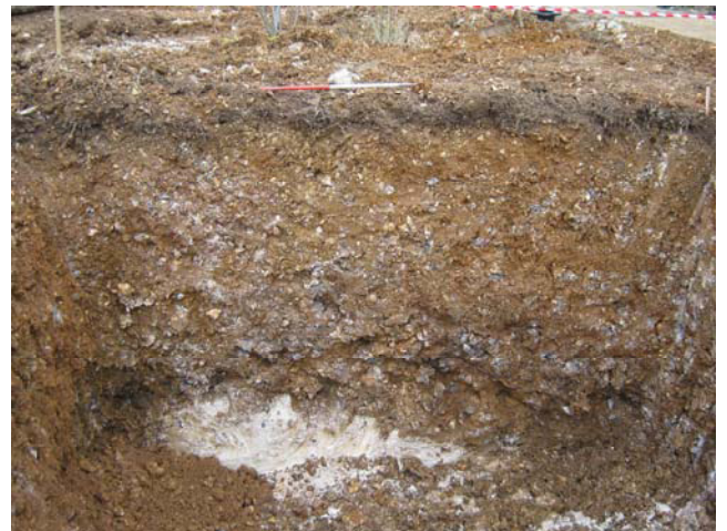
DP 12. Excavation for new soakway. Sample section 3. Looking north-east.
