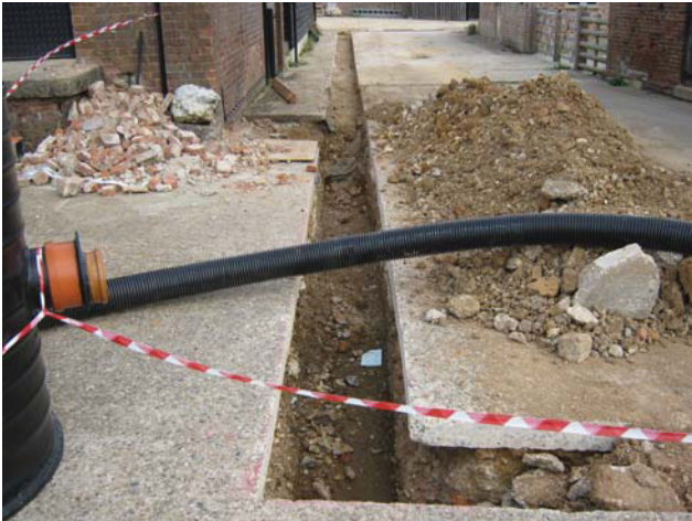
DP 3. Service trench to north-west of Maynes Cottage. Looking north-east.
