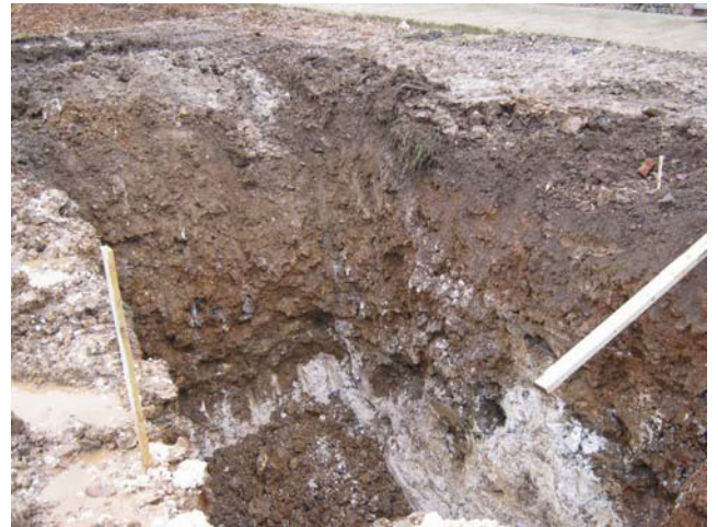
DP 8. Excavation for new biomass tank. Looking east.
