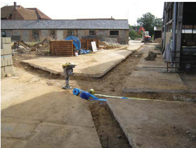
DP 5. Backfilled trenches in north part of the site. Looking south-east.
