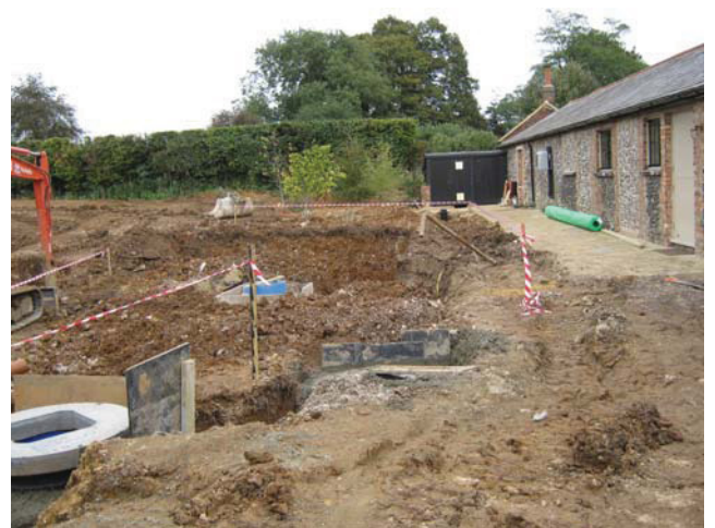
DP 10. Excavation for new soakway. Looking north-east.
