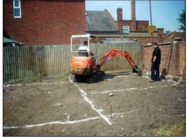
View of site with footings marked out
