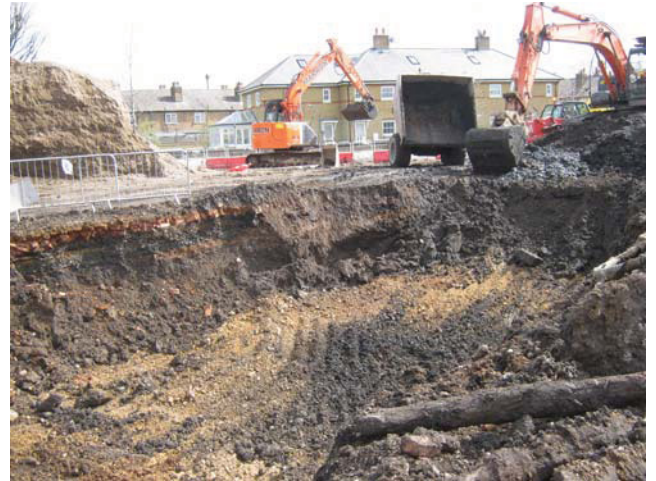
DP 14. Attenuation tank No 2. Looking east.
