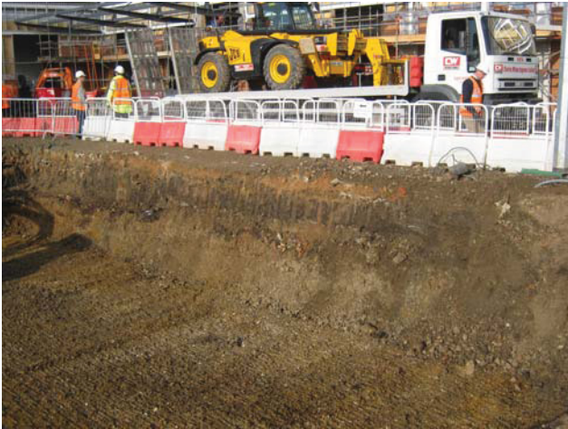
DP 13. Attenuation tank No 2. North-west side with sample section 3. Looking west.
