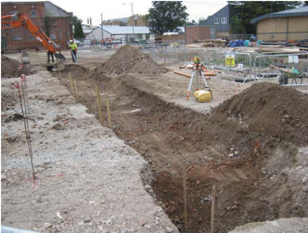
DP 3. Trench for foundation pads. Looking south-west.
