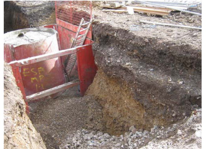
DP 4. Trench for foundation pads. Looking south-west.
