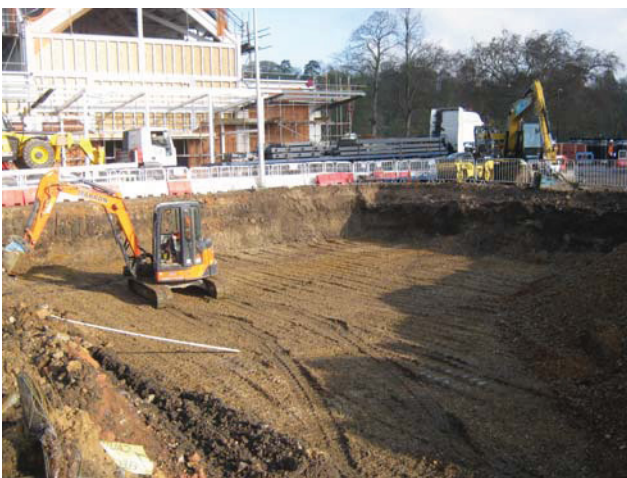
DP 11. Excavation for the southern attenuation tank (No 2). Looking north-north-west.
