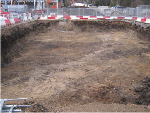
DP 7. Excavation for the northern attenuation tank (No 1). Looking north-west.
