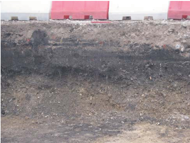
DP 9. Attenuation tank No 1. South-west side with sample section 3. Looking south-east.
