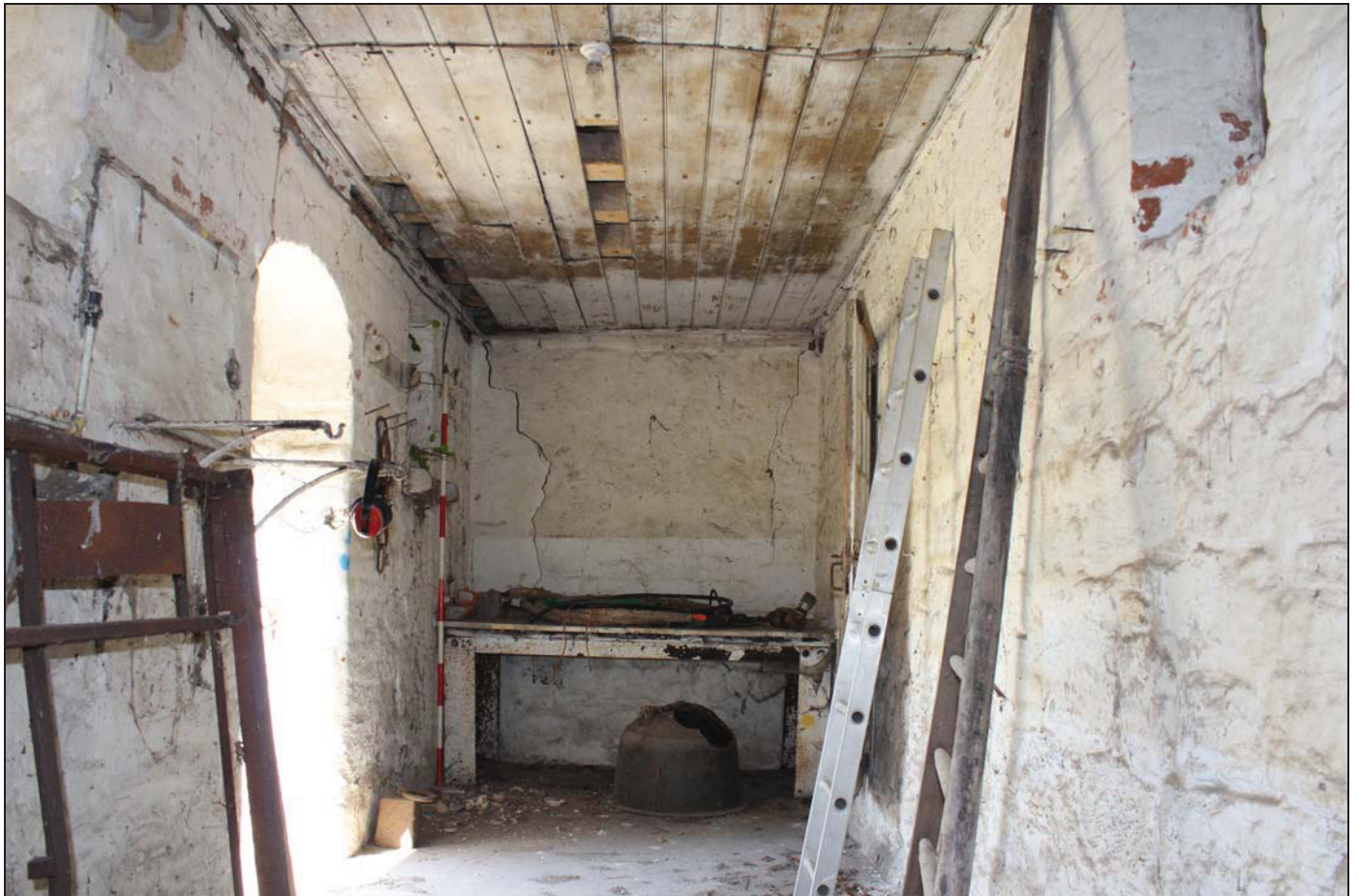
Plate 4 Room GF01, taken from the east (DP24)
