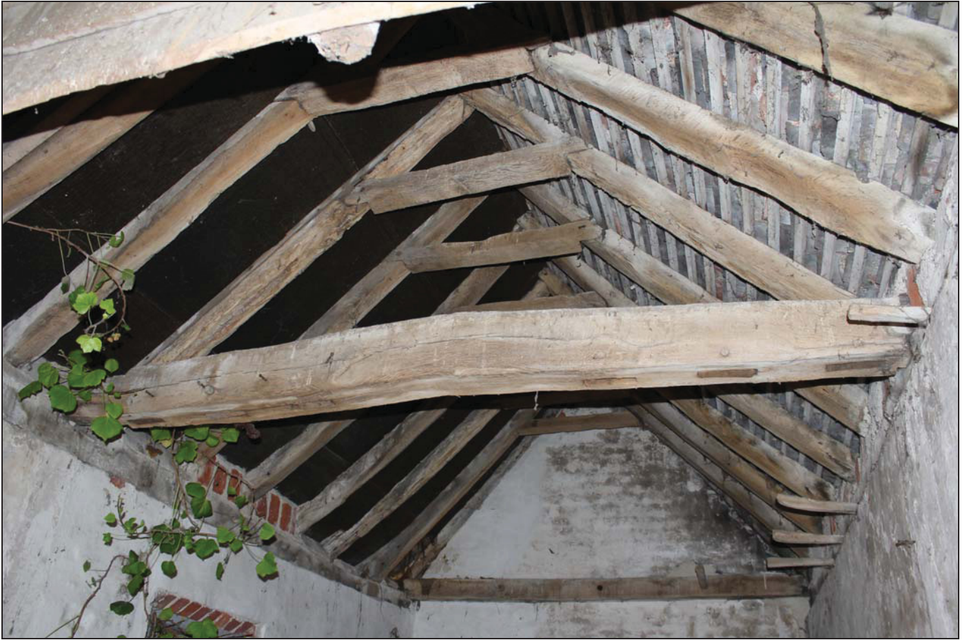
Plate 8 Roof structure over Room FF01, taken from the east (DP39)
