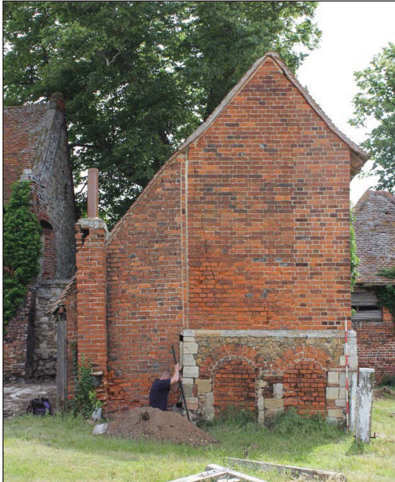
Plate 3 West elevation of the assessment structure, taken from the west (DP08)
