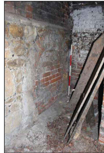
DP 28 Section of the north wall of the main body of the building showing a blocked archway at the west end enclosed by the lean-to, taken from the north-east
