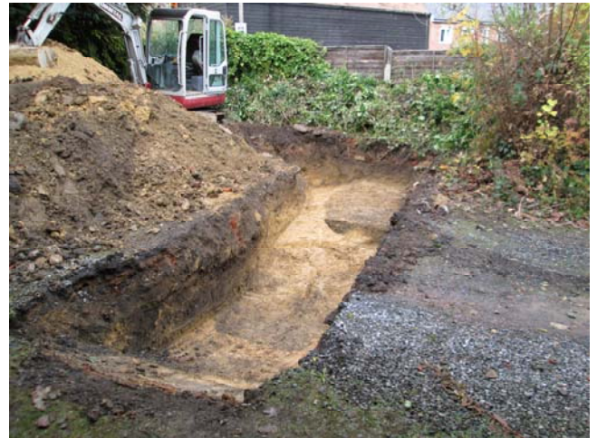
DP 2. Trench 1. Looking west-north-west.
