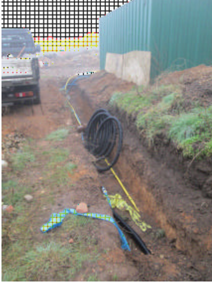
DP 13. Service trench. Looking south.
