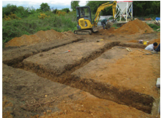
DP 10. Foundation trenches for annexe and garage. Looking north-west.
