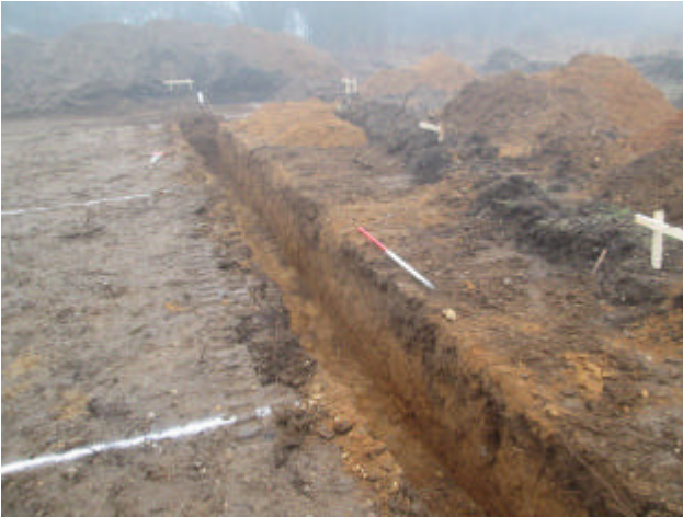
DP 3. South foundation trench. Looking south-east.
