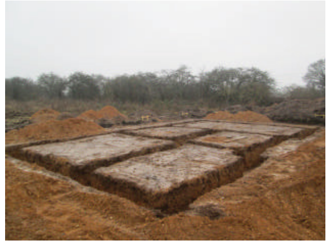
DP 2. Foundation trenches for new house. Looking south-west.
