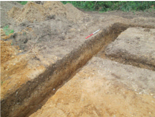
DP 11. South foundation trench for new garage. Looking south-west.
