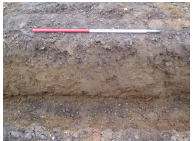
DP 6. West foundation trench. Sample section 2. Looking west-north-west.
