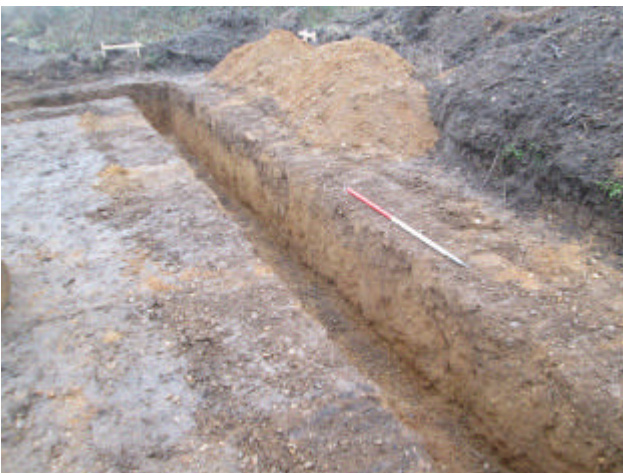
DP 5. West foundation trench. Looking south-west.
