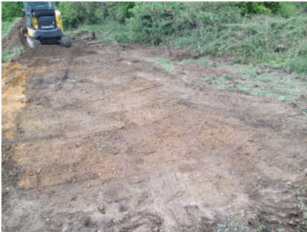
DP 9. Ground reduction within the area of new garage. Looking south-west.
