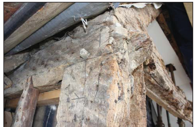
DP 50 View of the collar soffit showing wattle stave holes, taken from the west during monitoring
