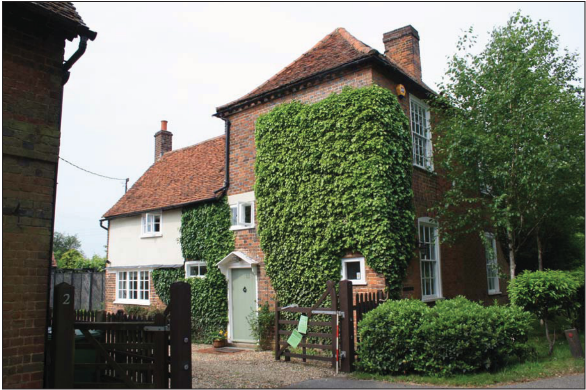
Plate 1 View of the house with front range and lower rear wing, taken from the north-east (DP 9)
