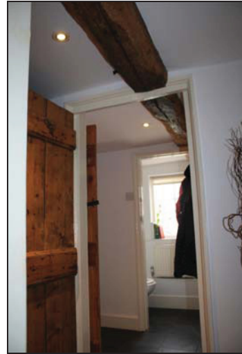
DP 20 View of the lobby area with WC to the rear, taken from the east
