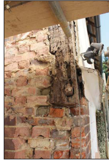
DP 42 Truncated and degraded south-east corner post, taken from the south during monitoring
