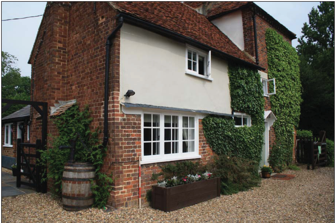
Plate 2 East elevation of the rear wing, taken from the south-east (DP 10)
