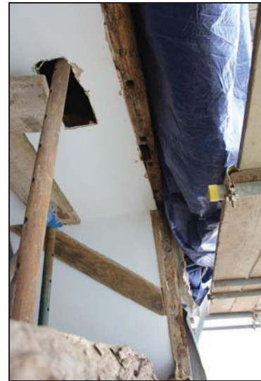
DP 50 View of the collar soffit showing wattle stave holes, taken from the west during monitoring
