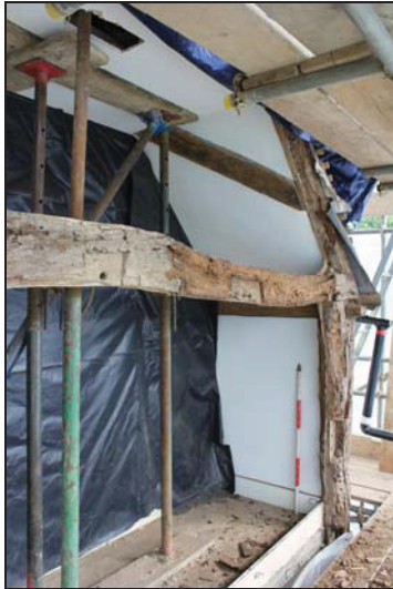
DP 47 Surviving principal timbers at first floor level, taken from the south-west during monitoring
