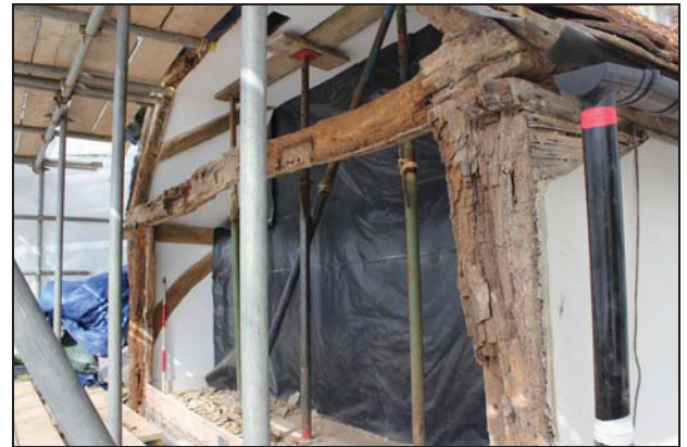
DP 42 Truncated and degraded south-east corner post, taken from the south during monitoring
