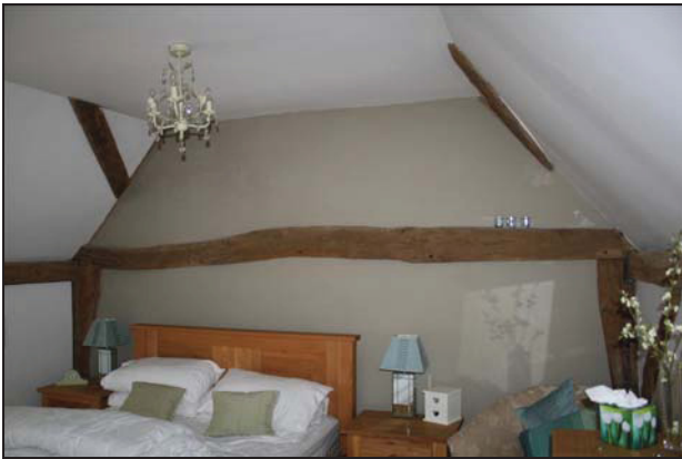
DP 19 Lamb's tongue chamfer stop on the bridging joist in the sitting room, taken from the north-east
