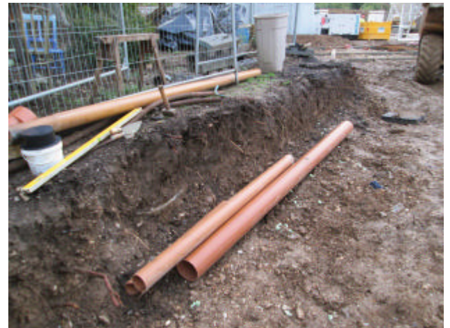
DP 16. Northern part of the site. Looking east.
