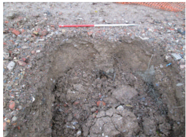
DP 18. Foundation pit in western part of the site. Sample section 4. Looking west-north-west.
