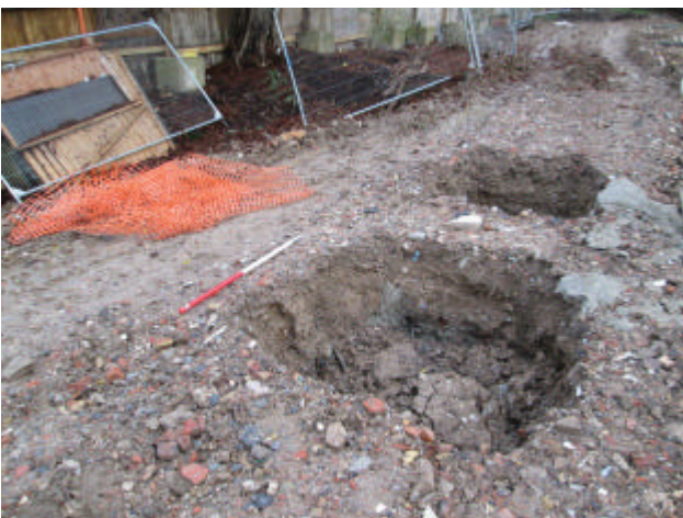
DP 17. Foundation pits in western part of the site. Looking north.
