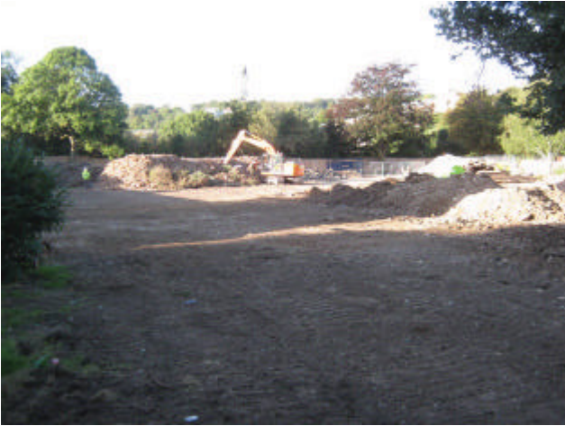
DP 1. The site during demolition works. Looking south-south-west.
