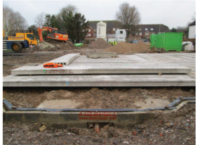
DP 22. Foundations in southern part of the site. Looking north-north-east.
