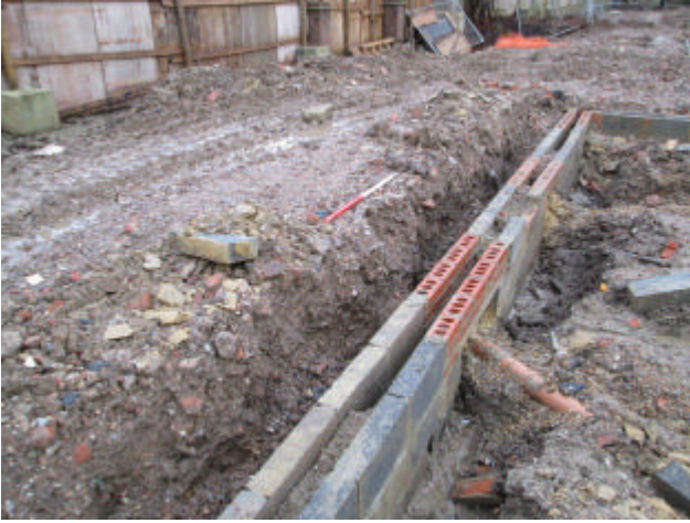
DP 7. Foundations in western part of the site. Looking north.
