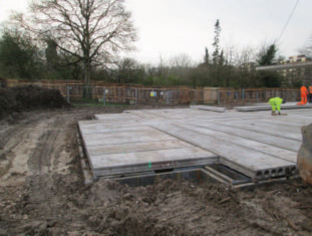
DP 21. Construction works in southern part of the site. Looking south-south-west.
