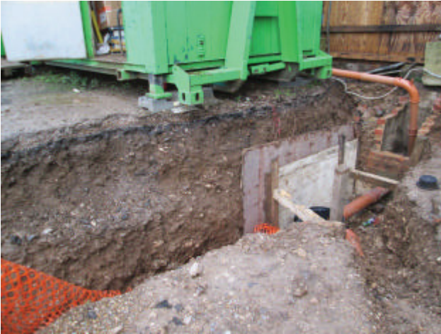
DP 13. Excavations in north-western part of the site. Looking north-north-west.
