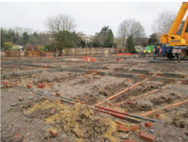
DP 5. The site with new foundations. Looking north-north-west.
