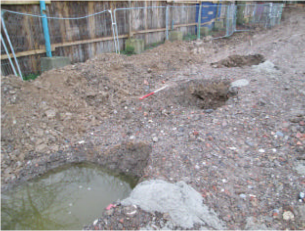
DP 19. Foundation pits in southern part of the site. Looking south-west.
