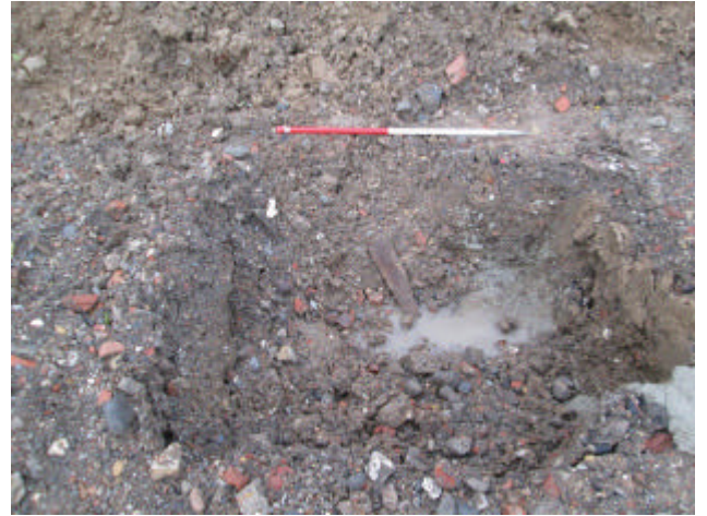
DP 20. Foundation pit in southern part of the site. Sample section 5. Looking south-south-west.
