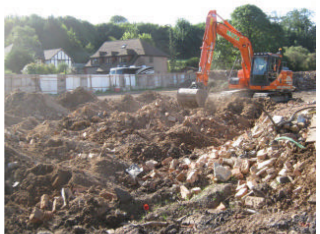
DP 2. Demolition works. Looking south-south-east.
