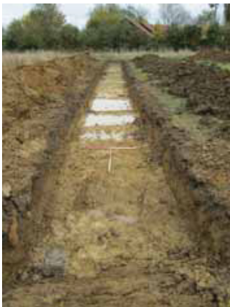
3 Trench 2. Looking north-east.
