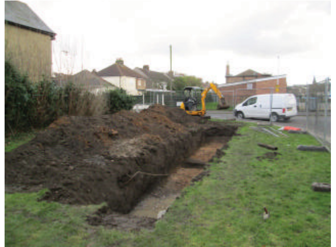
DP 2. The site with Trench 1. Looking south-south-east.
