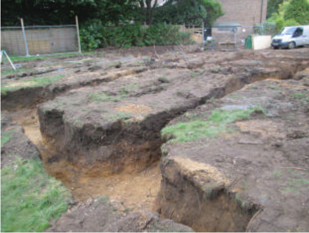
DP 7. South/central foundation trenches area. Looking north.
