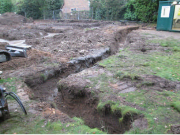
DP 13. Trench for new retaining wall. Looking east.
