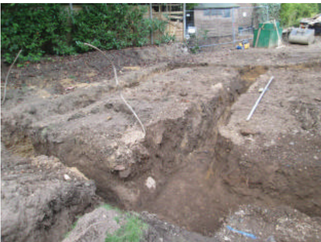
DP 5. West foundation trenches area. Looking north.
