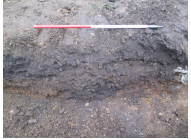
DP 14. Trench for retaining wall. Sample section 7. Looking south.
