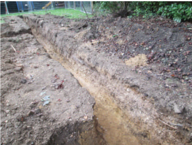
DP 3. West foundation trench. Looking south-west.
