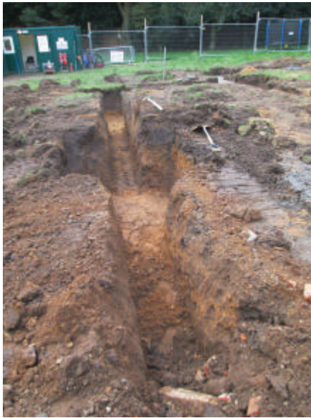
DP 9. Central foundation trench. Looking south-south-west.
