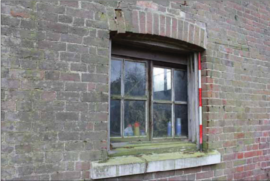
DP 7 Original sash windows removed and replaced with casements, north-west elevation, taken from the north
