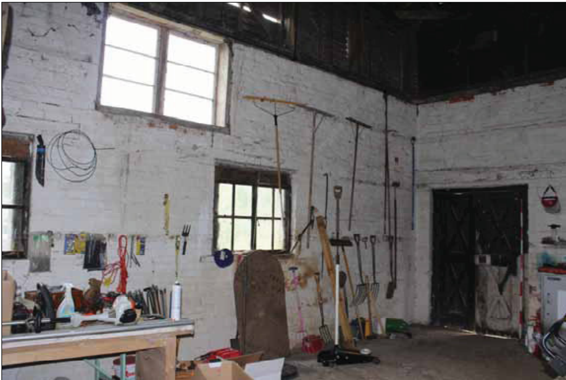
DP 12 Interior, north-east end of the building, taken from the south
