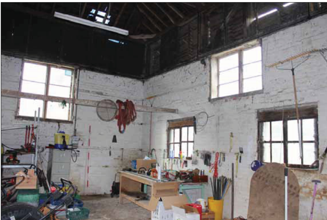
DP 14 Interior, south-west end of the building, taken from the east
