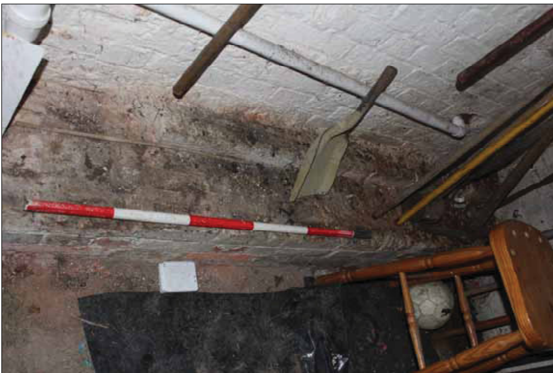
DP 16 Low brick plinth against north-east wall, taken from the north-west
