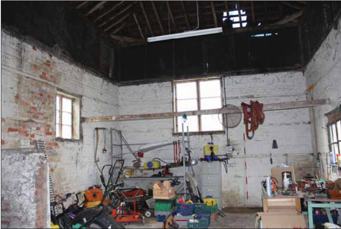
DP 13 Interior, south-west end of the building, taken from the north-east
