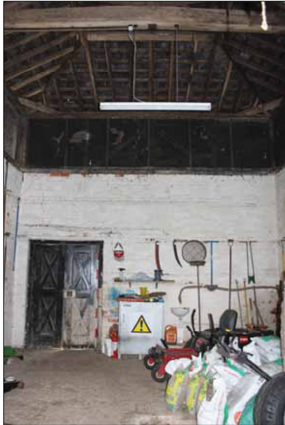
DP 11 Interior, north-east end of the building, taken from the south-west
