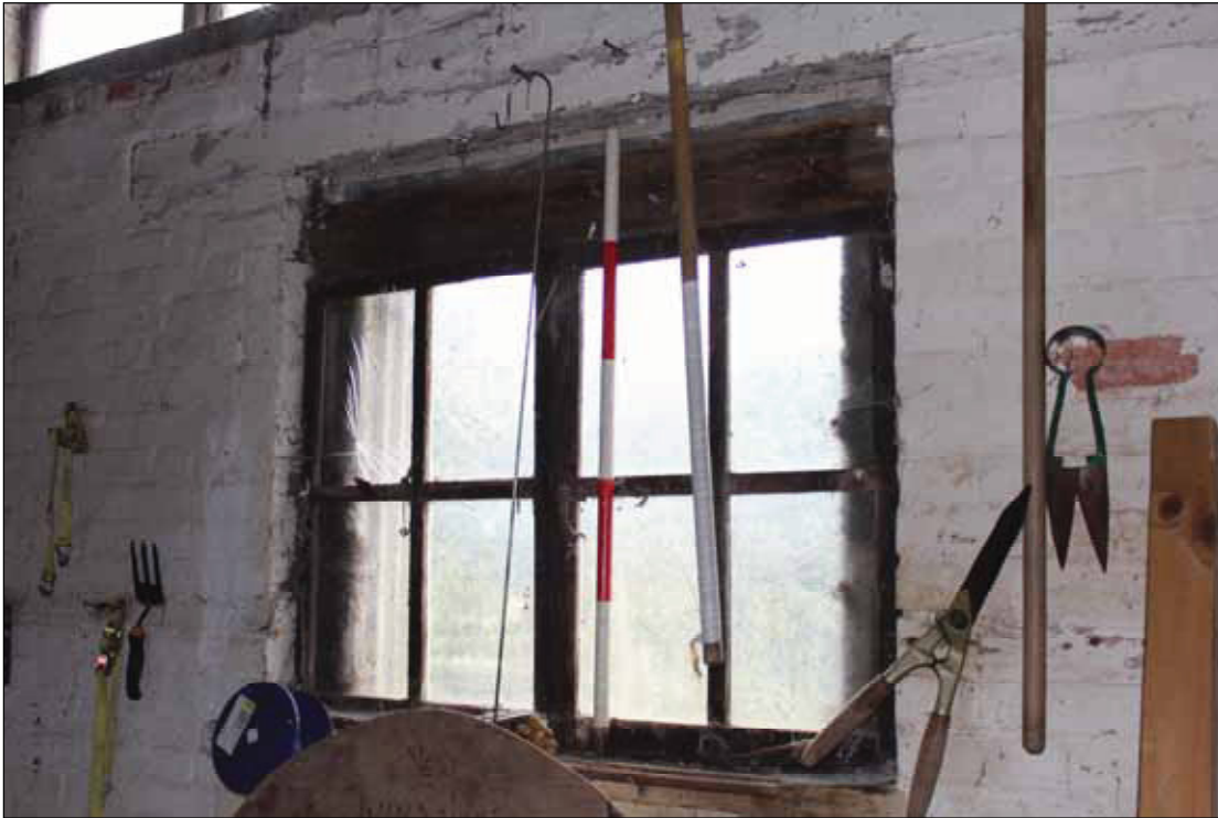
DP 17 Later casement windows fitted from the inside, north-west elevation, taken from the east
