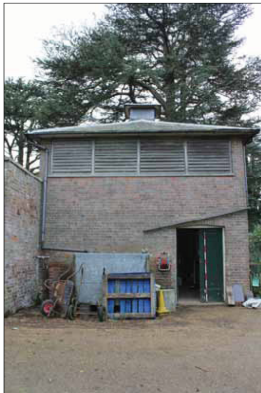
DP 2 North-east elevation, taken from the north-east
