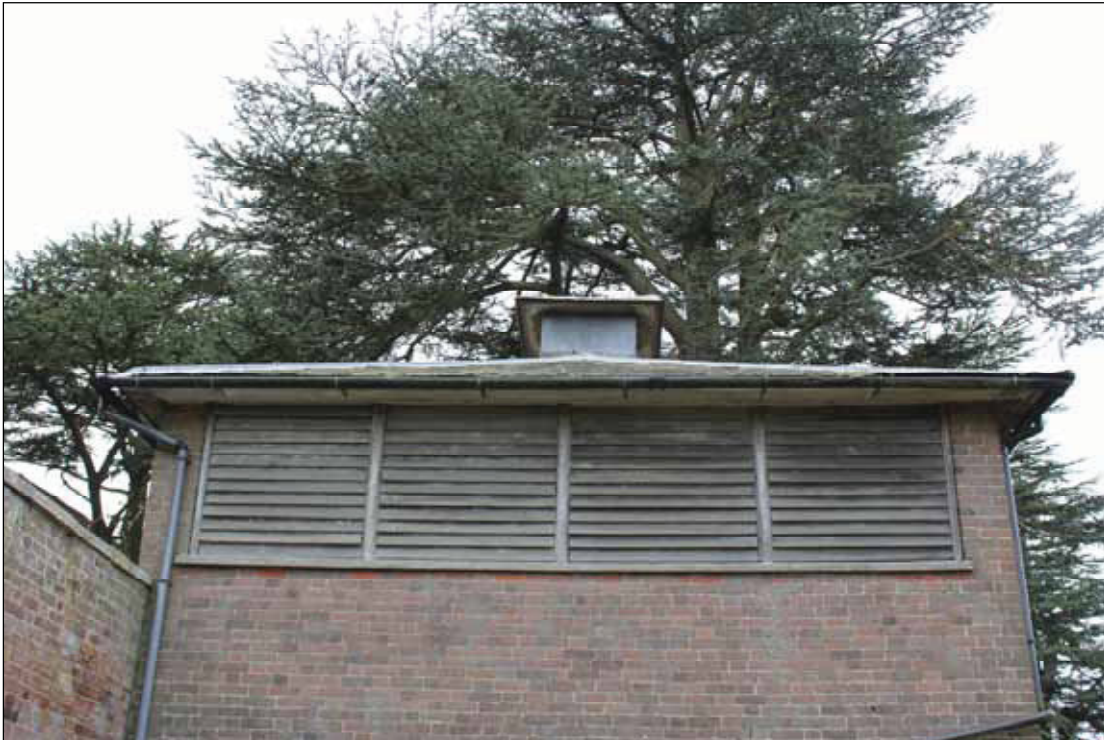
DP 3 Ventilation apertures at high level, north-east elevation, taken from the north-east
