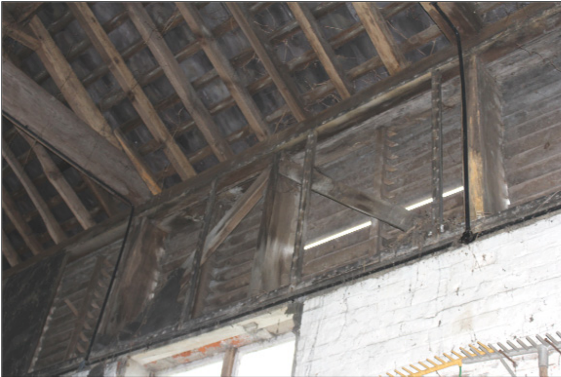
DP 23 Upper ventilation louvres, taken from the east
