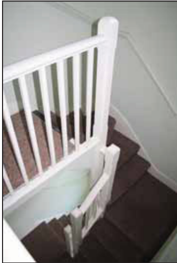
DP 67 Staircase in the south-east area of the 1900 range (first floor), taken from the south-east
