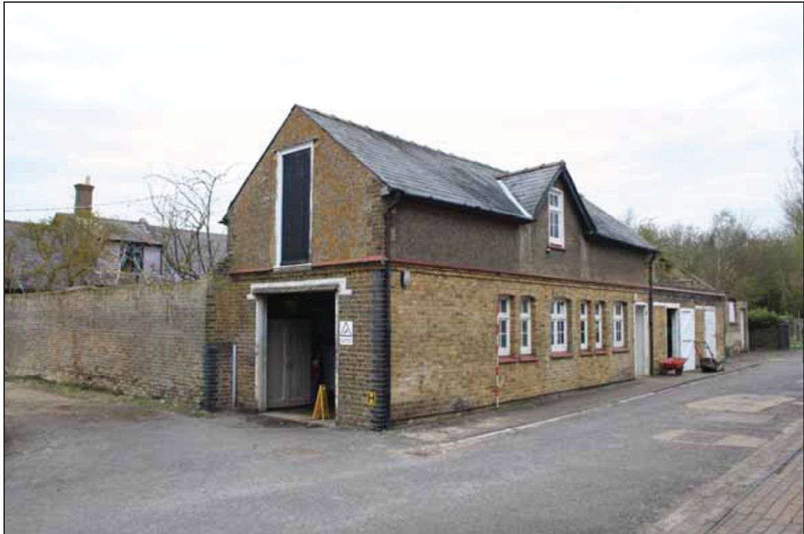
Plate 13 South and east sides of Outbuilding 2, taken from the south-east (DP 31)
