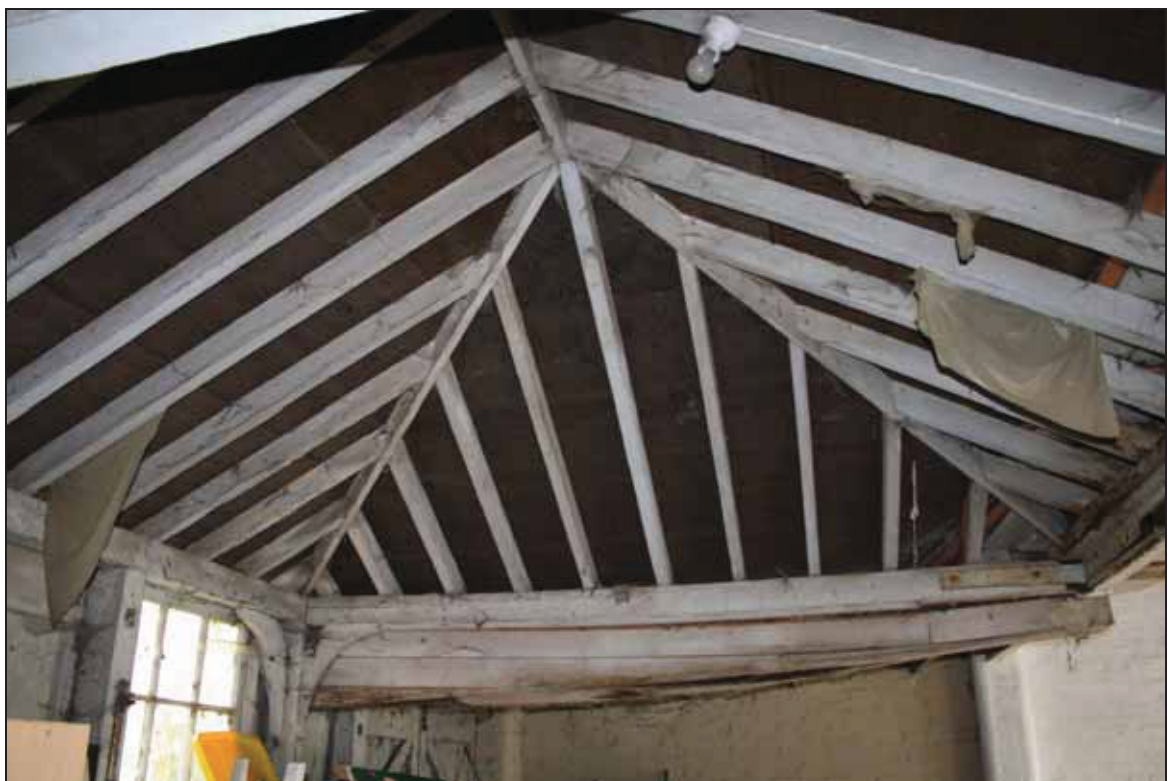
Plate 12 South-west roof structure of Outbuilding 1, taken from the south (DP 26)
