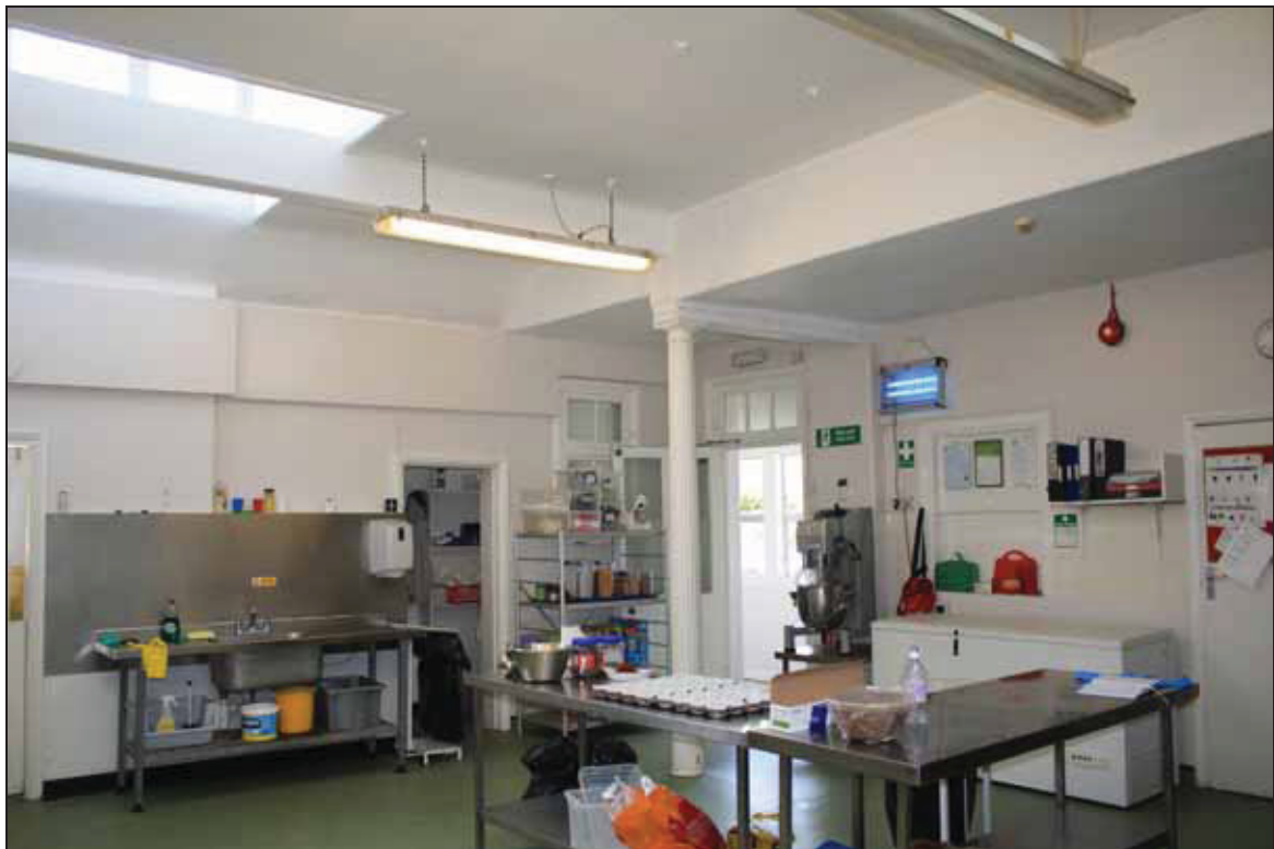
Plate 6 Kitchen in the 1900 range which appropriates part of the earlier north range, taken from the south-east (DP 47)
