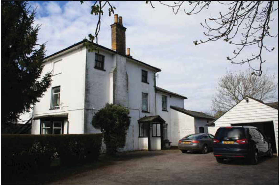
Plate 1 North side of the north range, taken from the north-east (DP 08)
