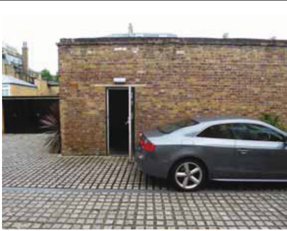
5. Looking west from Hazlewood Mews at the rear (eastern) entrance to the site (the brick building)
