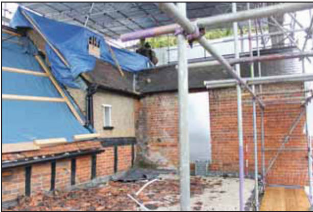
Remains of timber-framing to the rear elevation seen between corridor extension and flat roofed extension, taken from the west
