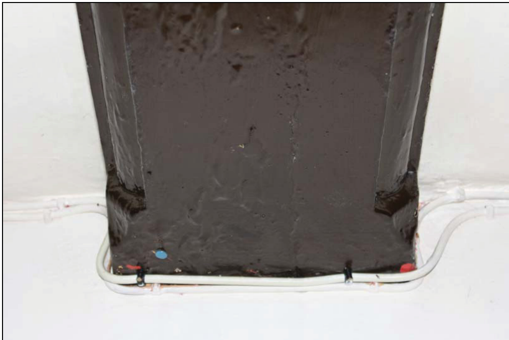
Plate 10 Lamb's tongue chamfer stops to the binding joist, GF02, taken from the north (DP 23)
