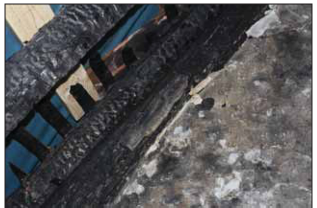
Surviving king strut at partition between FF05 & FF06, taken from the north-west
