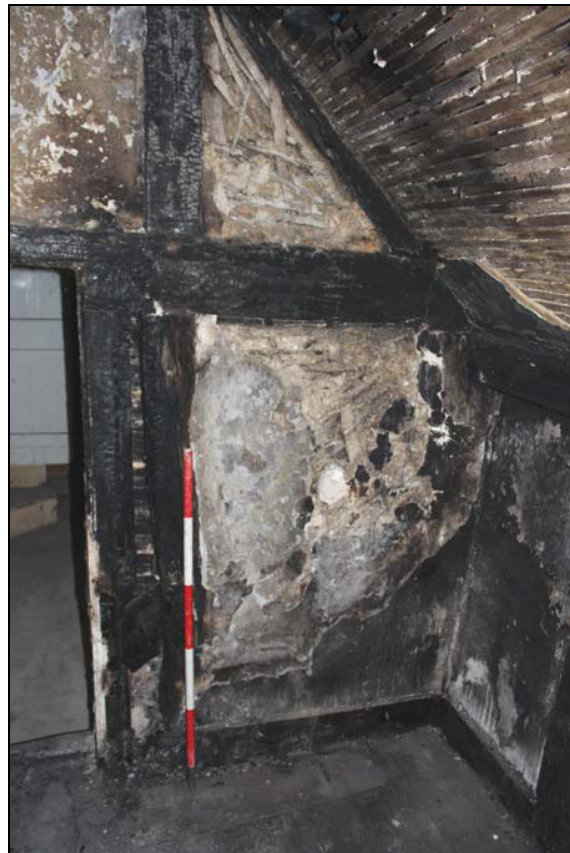
Plate 14 Wattle and daub panels to the south elevation, FF03, taken from the north-east (DP 72)
