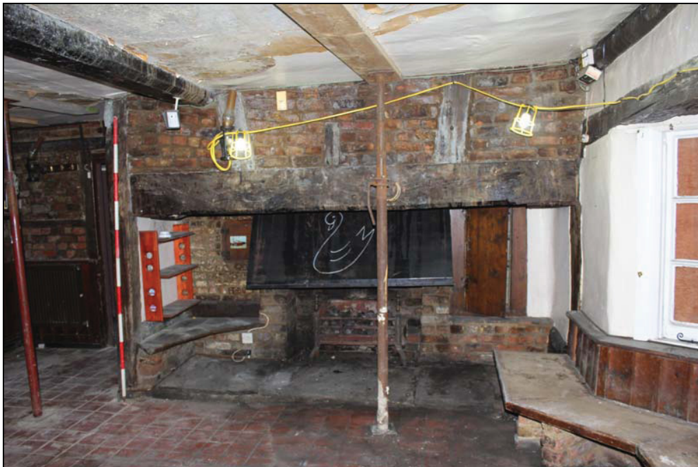
Plate 8 Large inglenook fireplace, GF01, taken from the south-east (DP 30)
