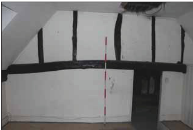
Timber framed partition between FF05 & FF06, taken from the south-east
