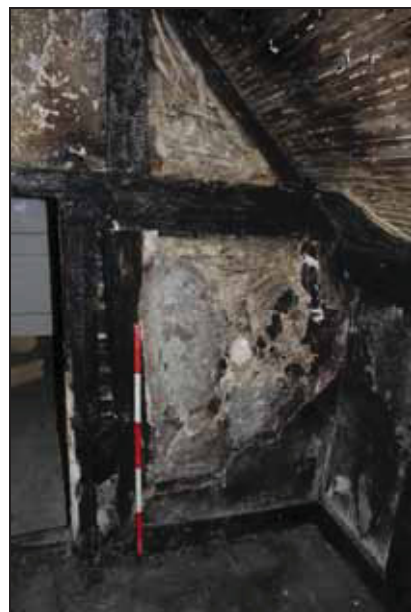
Charred intermediate collars and common-rafters, FF03, taken from the north-west
