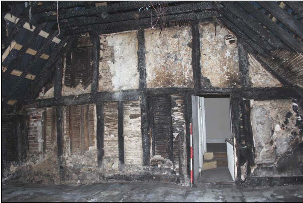
Plate 13 South elevation, FF03, taken from the north (DP 67)
