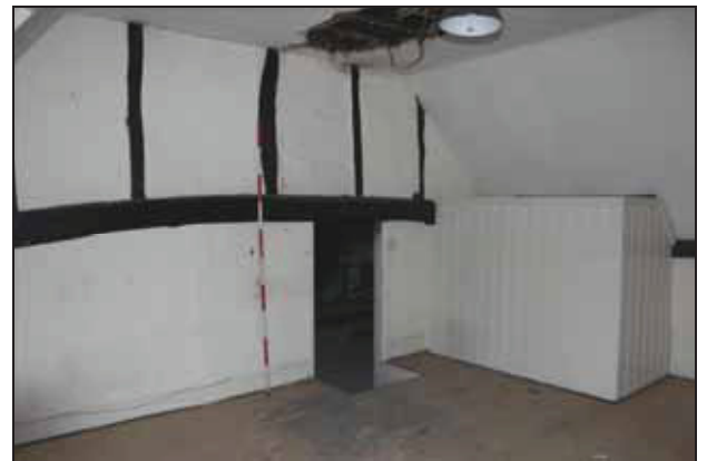
Timber framed partition between FF05 & FF06, taken from the north-east
