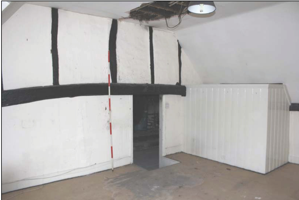
Plate 16 Timber framed partition between FF05 & FF06, taken from the north-east (DP 84)
