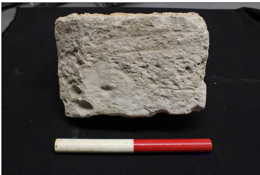
4 Side elevation of worked stone piece 1 with plain chamfer on the left
