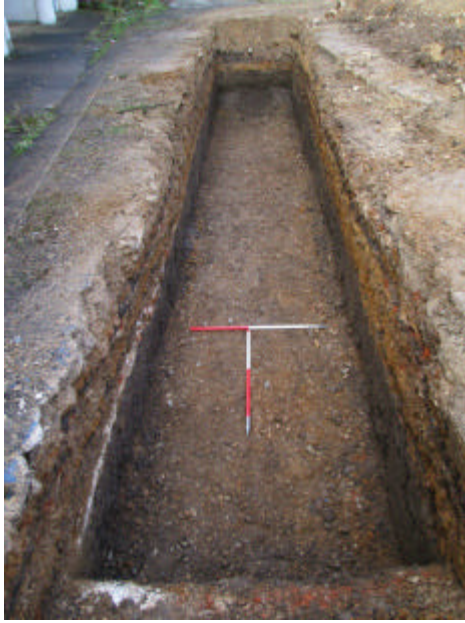
DP 7. Trench 2. Looking north-north-west.
