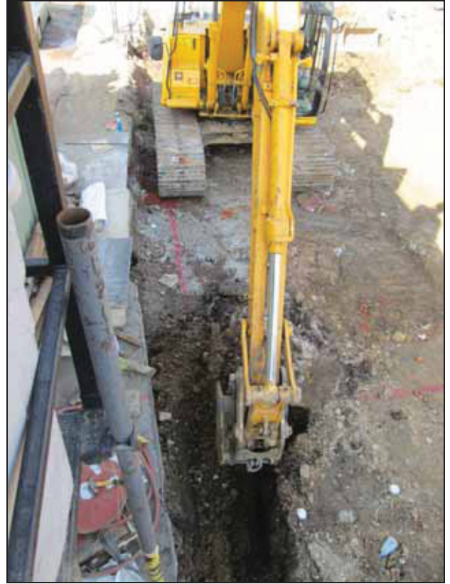
Footings being excavated
