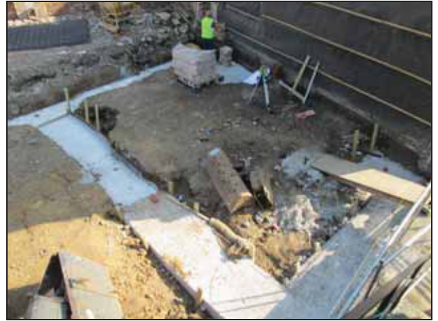
Footings being excavated
