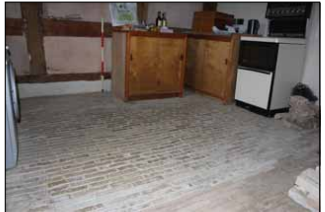
10 General view of the floor (eastern service-wing), facing south-west
