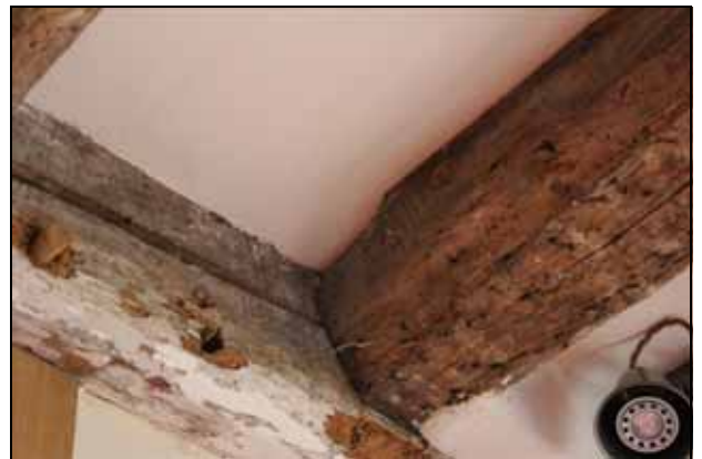
Detail of scribed assembly marks in binding joist and ceiling joist, facing north-east
