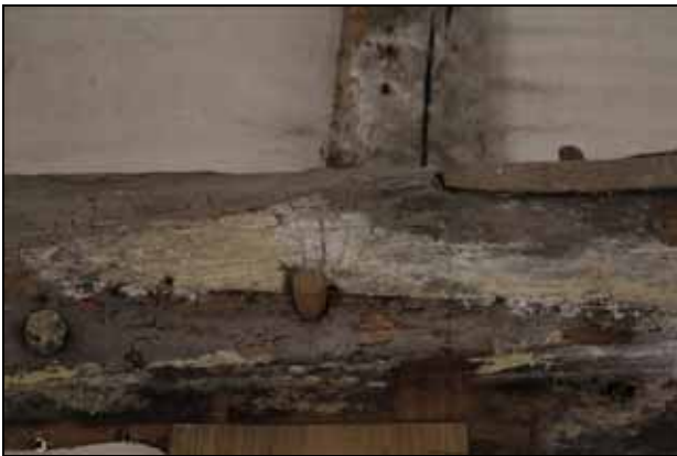
Detail of scribed assembly marks, facing south
