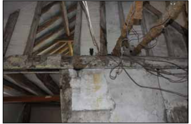
Detail of the binding joist showing sawn off floor joists (left) and blank area to east marking aperture in original ceiling of this bay, facing south
