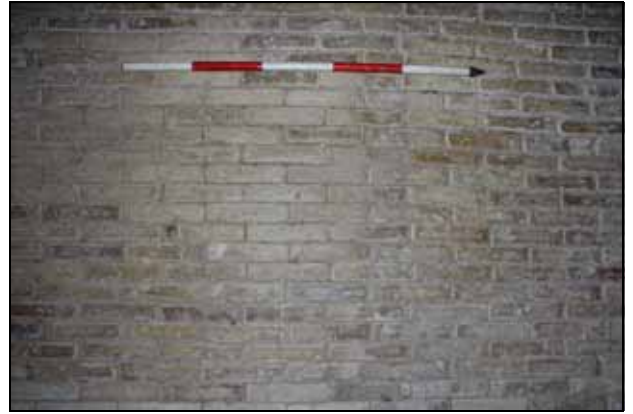
8 Typical sample of the brickwork of the paviour floor (eastern service-wing), facing south
