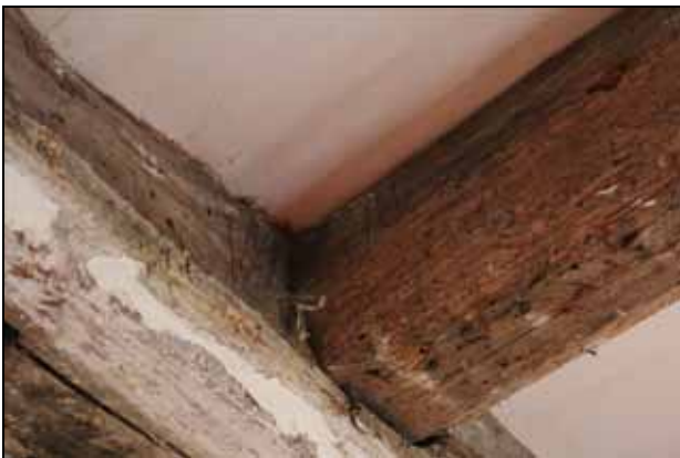
Detail of scribed assembly marks in binding joist and ceiling joist, facing north-east
