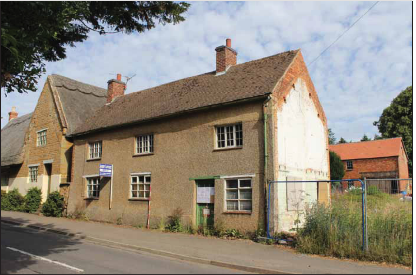
Plate 1 South elevation of the house, taken from the south-east (DP02)
