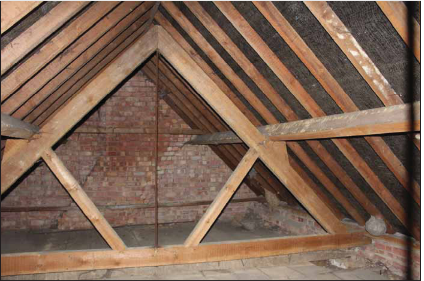
Plate 9 Later double-framed roof structure, taken from the east (DP78)
