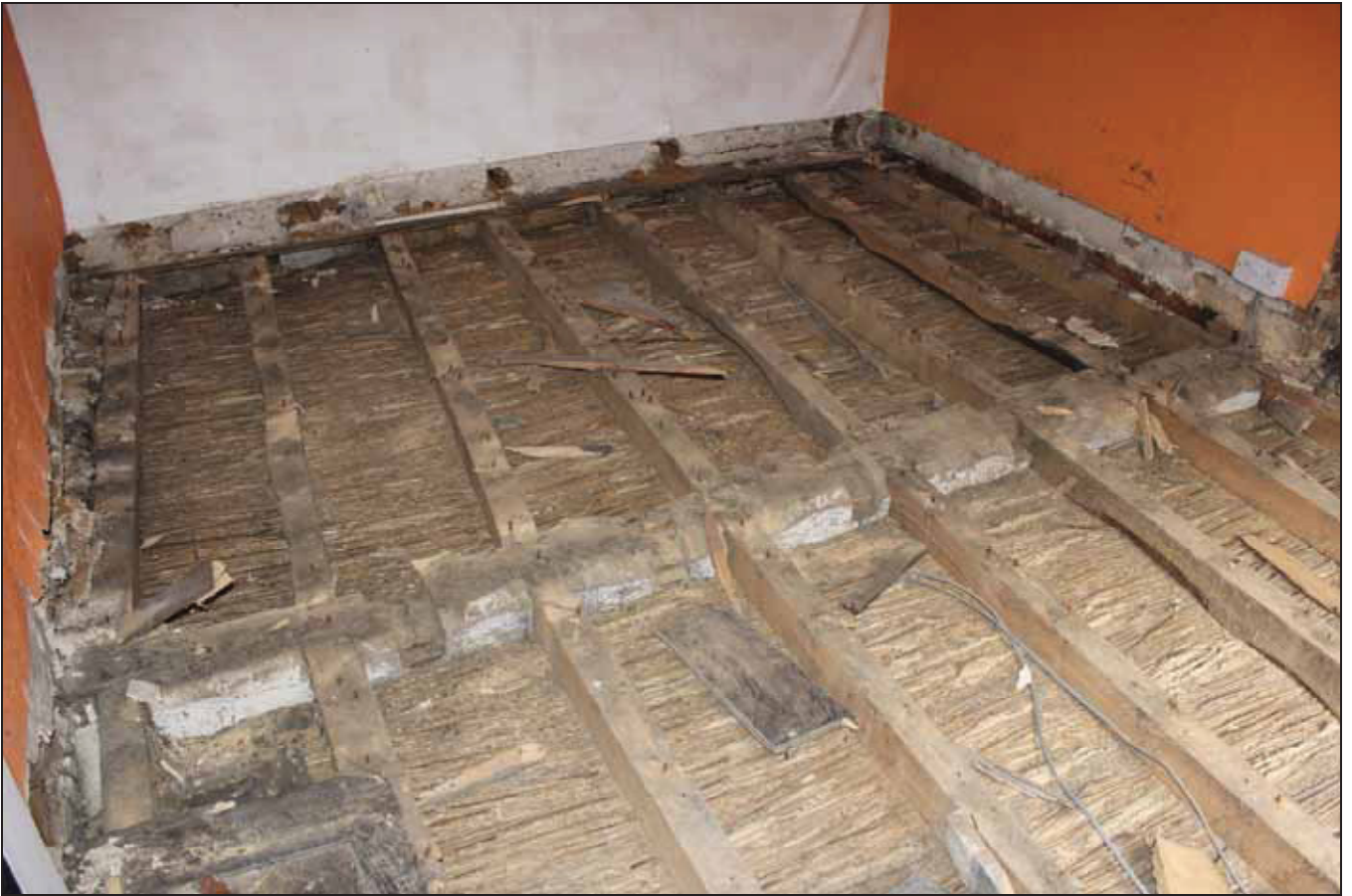
Plate 5 Exposed floor structure in Room FF02, taken from the south-east (DP62)
