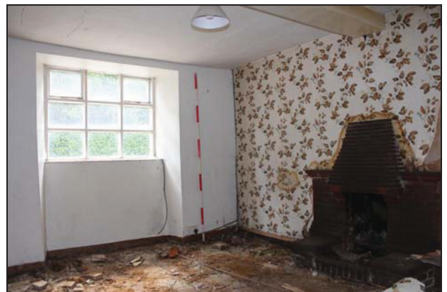
DP 24 South-west area of Room GF01, taken from the north-east
