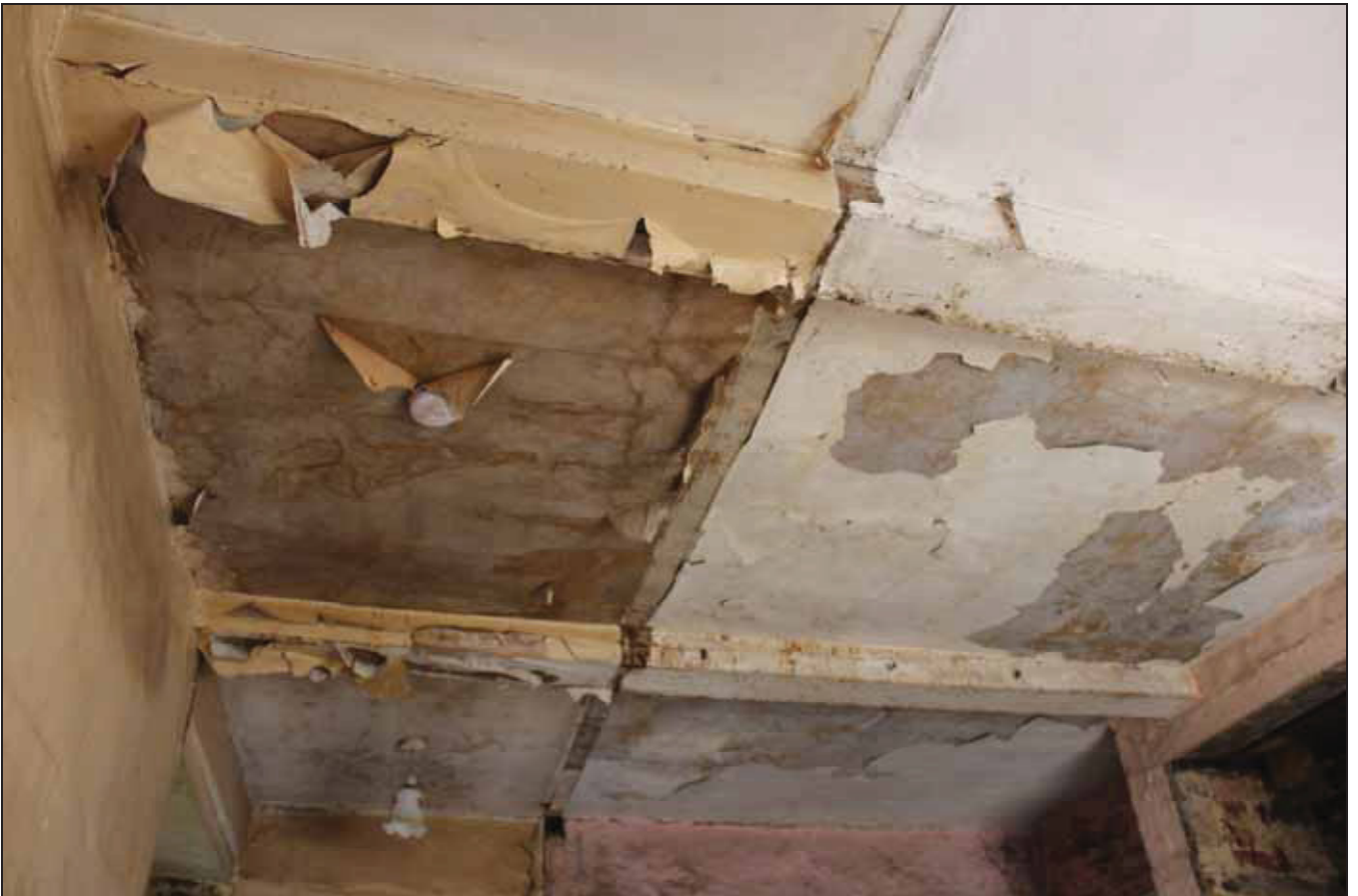
Plate 4 Ceiling of Room GF03, taken from the south-west (DP36)
