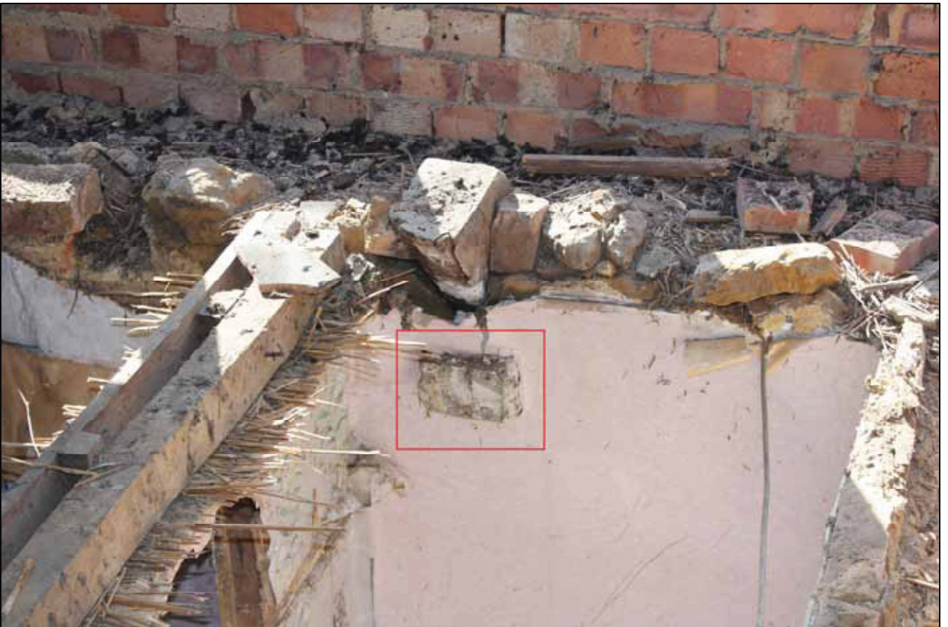
Plate 10 Evidence in the cupboard (FF03) showing stumps of the original tie-beam (indicated) and principal rafter, taken during demolition from the north
