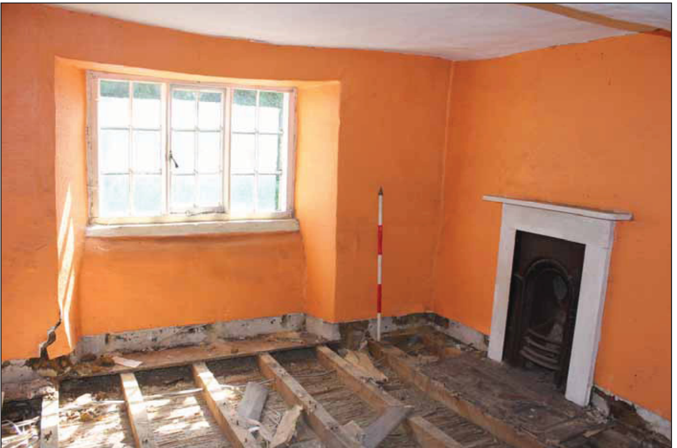
Plate 6 Room FF02, taken from the north-east (DP57)
